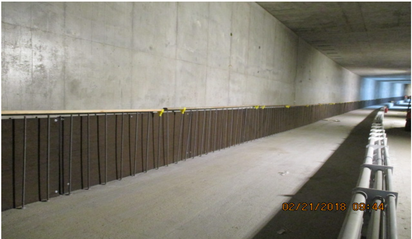
UG4 – Installation of epoxy rebar dowels for SB emergency walkway.
