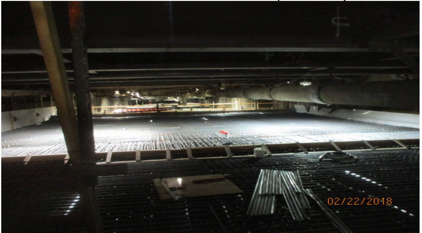
LEIMERT PARK STATION - Preparing roof section for concrete placement.
