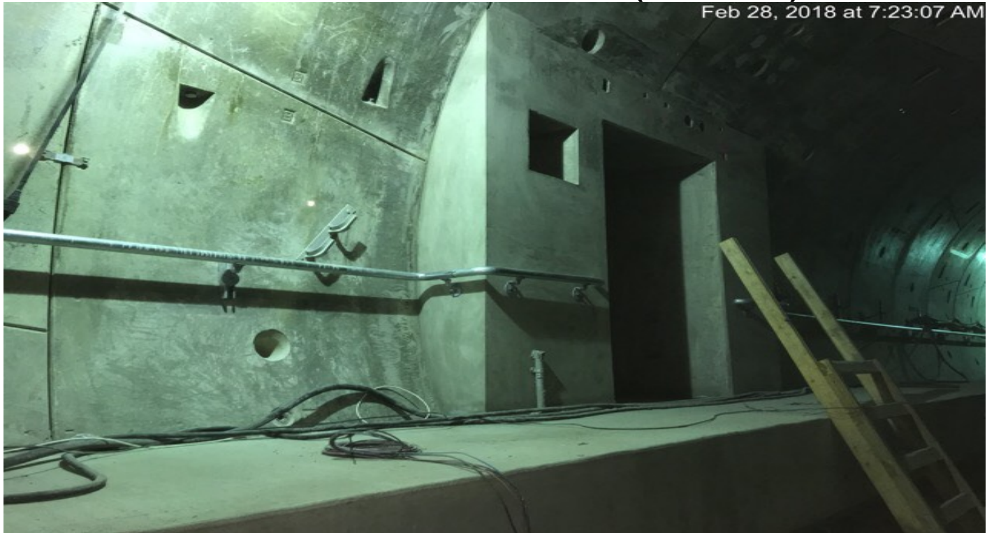
TUNNELING – Installing handrail adjacent to CP-4.
