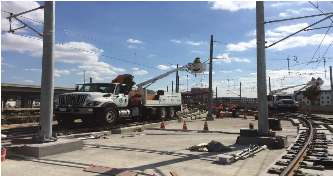
GREENLINE TIE-IN - Installing overhead catenary system.
