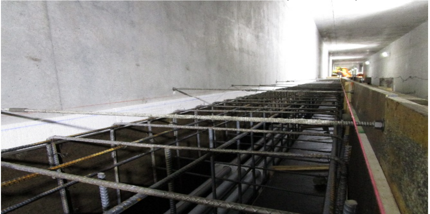
UG#3 - Installation of formwork for NB emergency walkway.
