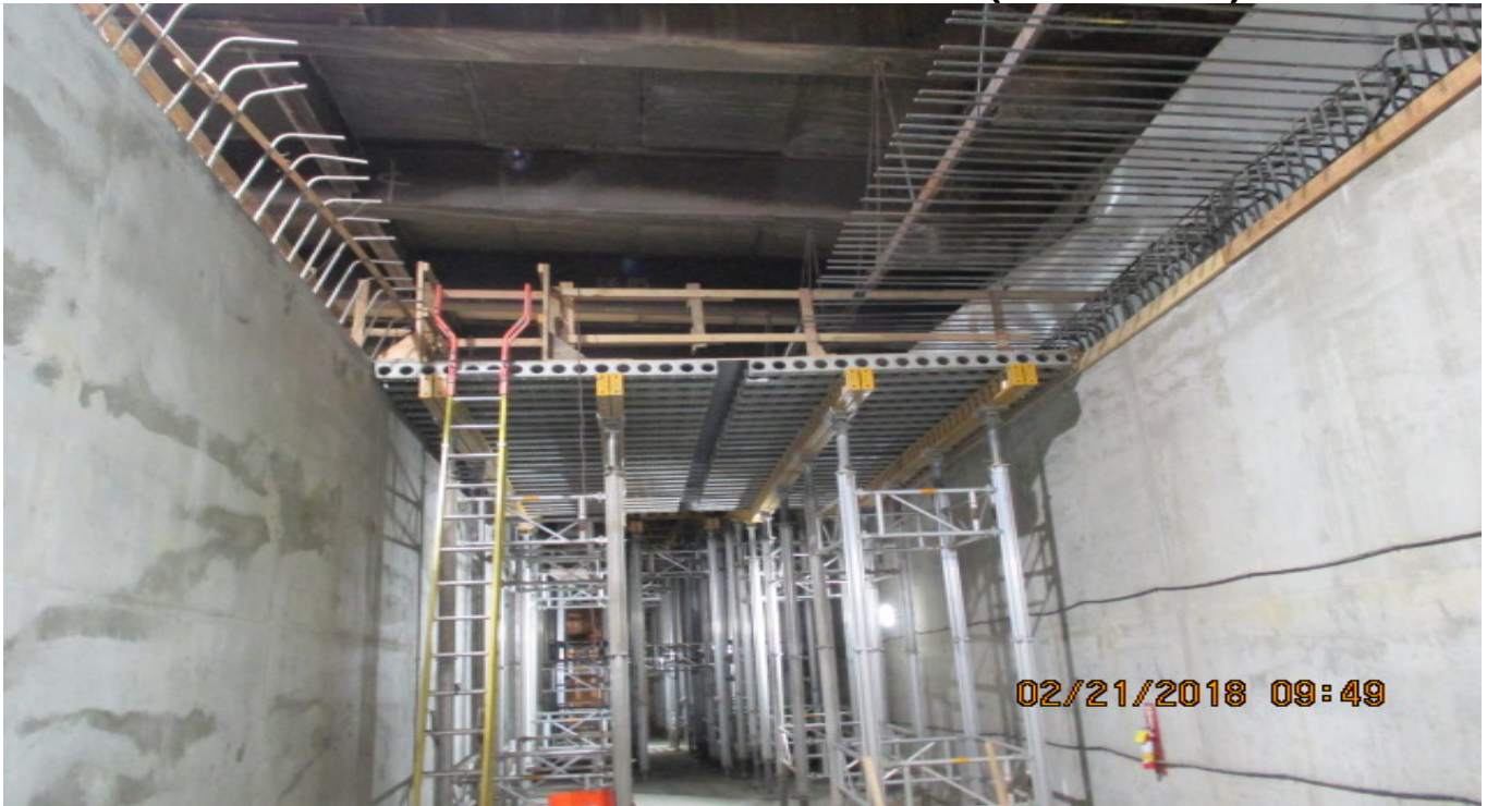
UG4 – Installation of falsework for roof deck.
