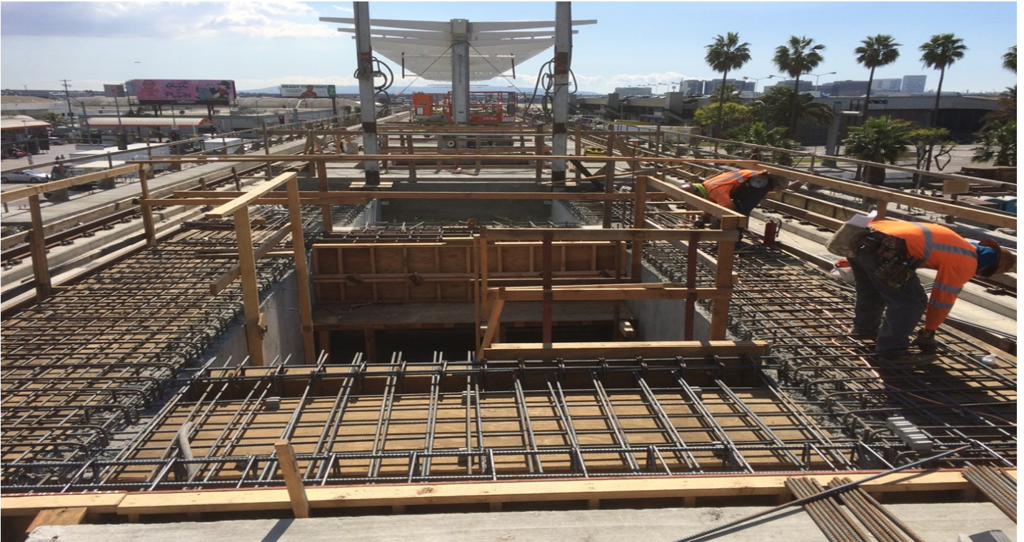
AVIATION/CENTURY STATION – Platform rebar installation at the service building exit corridor.
