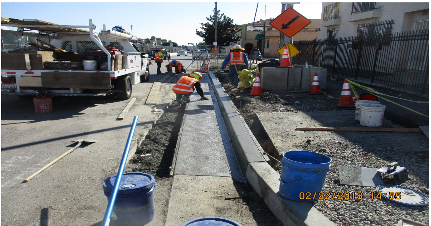
PARK MESA - Placement of curb and gutter at 59th street.
