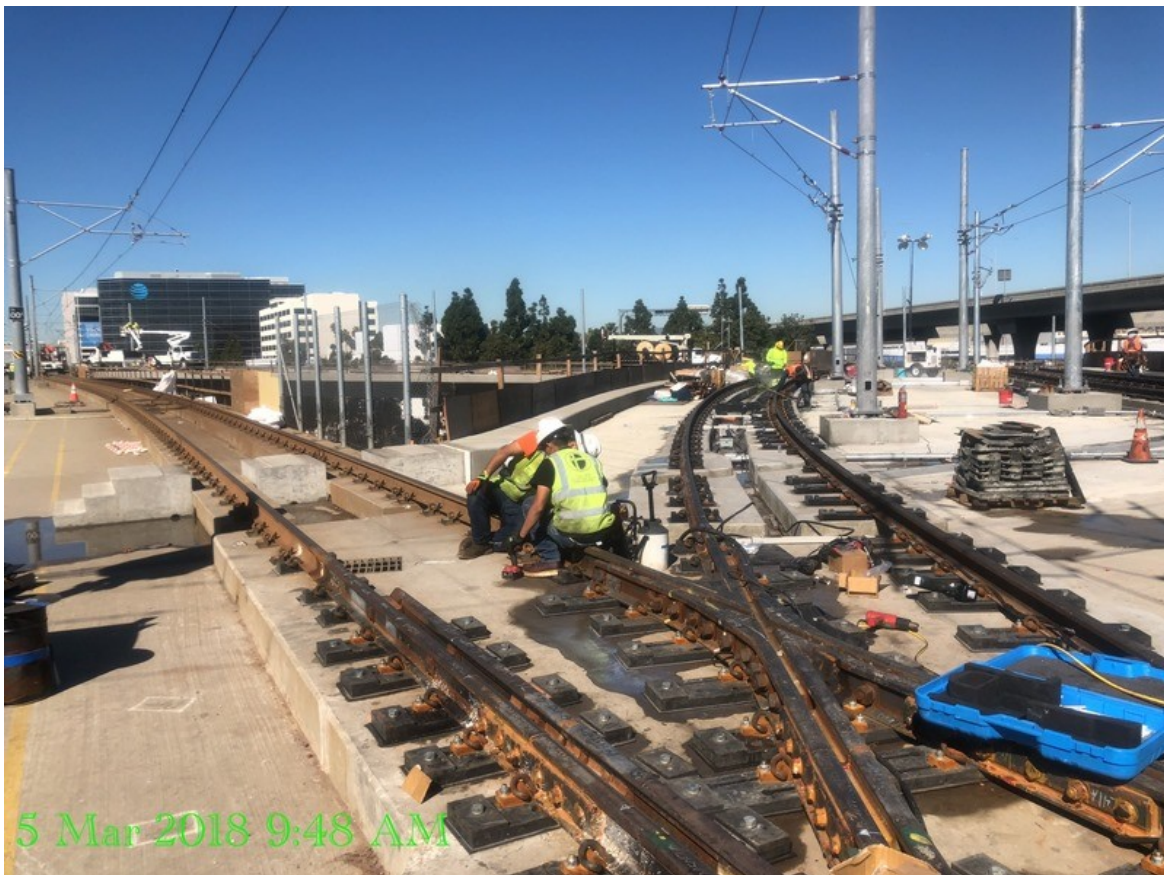
GREENLINE TIE-IN – Trackwork and overhead catenary system installation.
