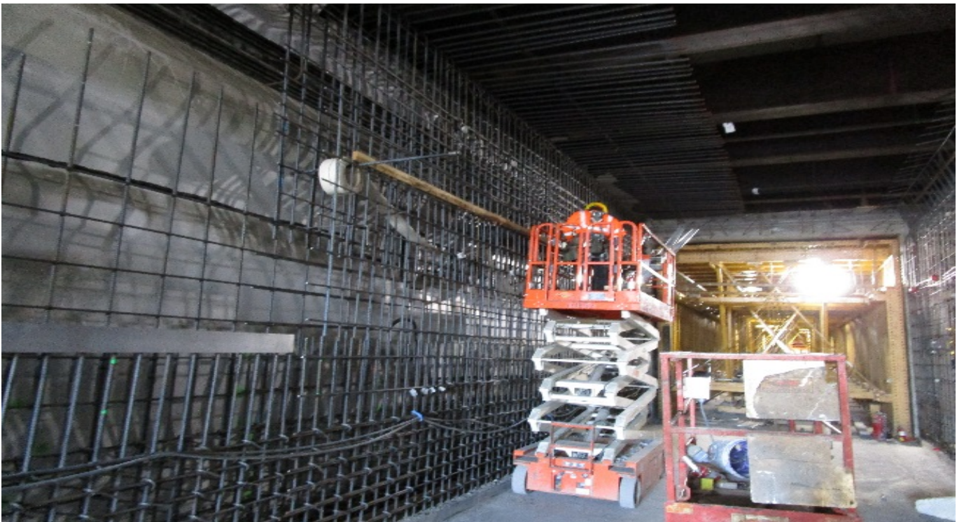
UG#3 - Installation of rebar for center wall.
