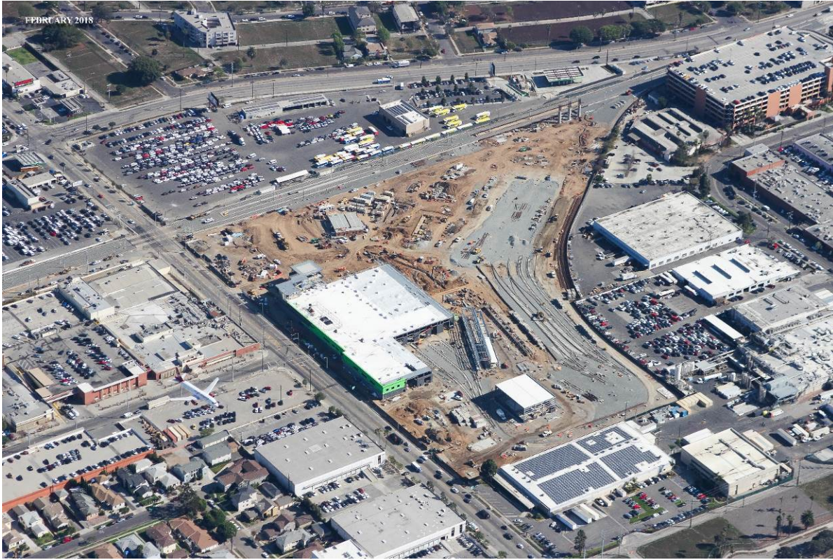
SOUTHWESTERN YARD – Aerial photo as of March 2, 2018.
