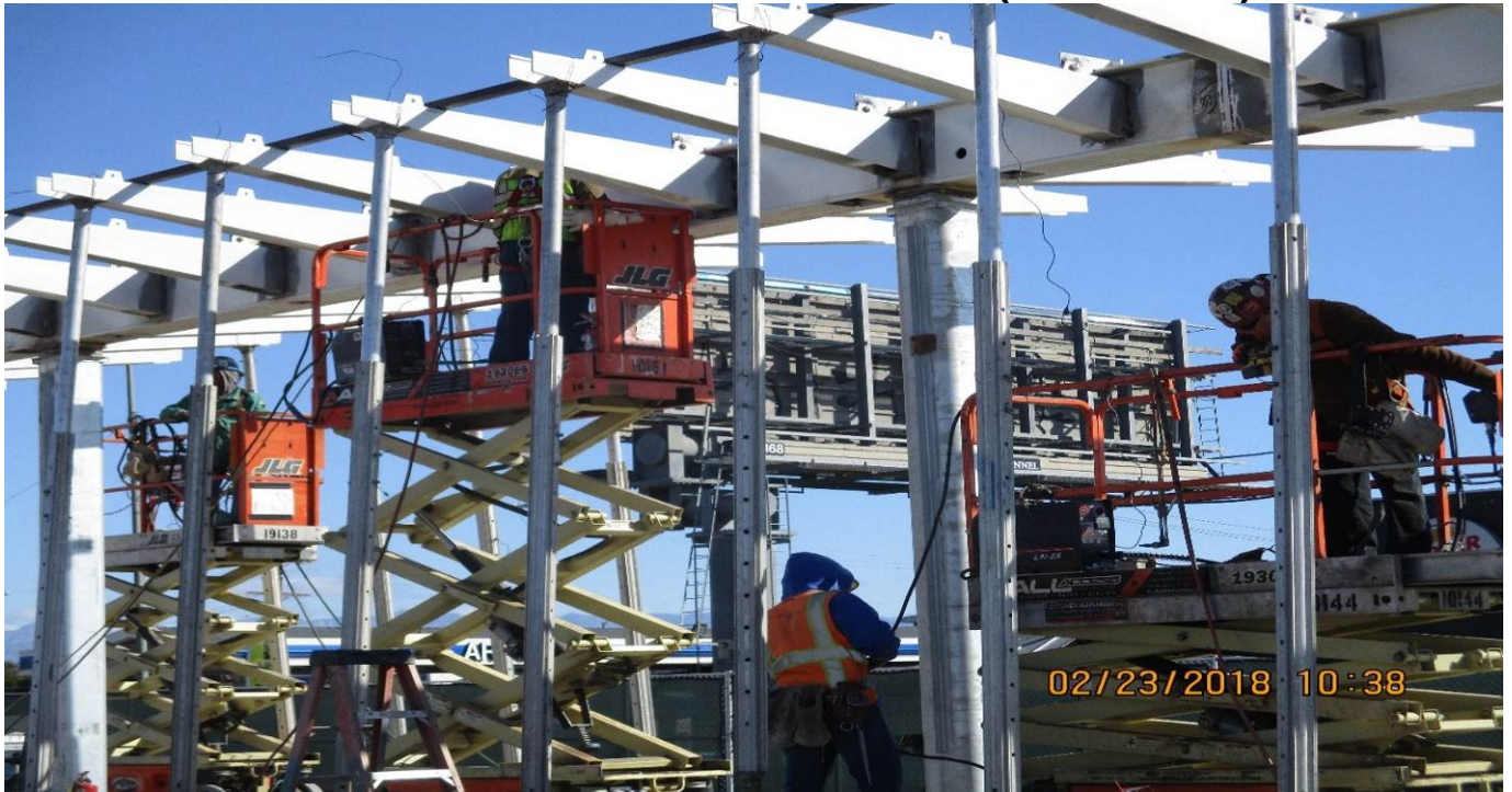
HYDE PARK STATION - Welding canopy.
