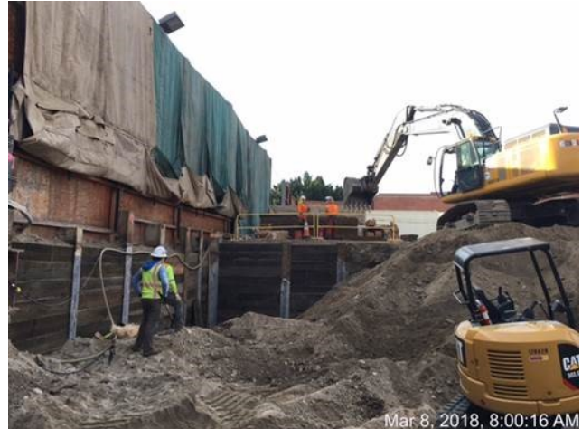
Excavation for Central Station and Wye
