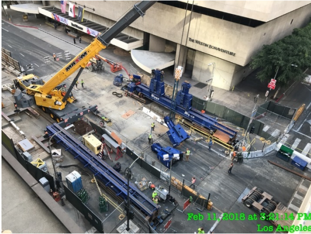
Gantry Crane demobilization
