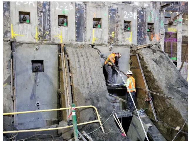
LA Times Building underpinning
