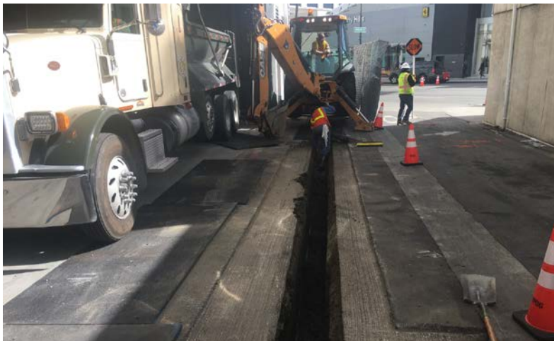
SCG Utility Work in Beverly Hills
