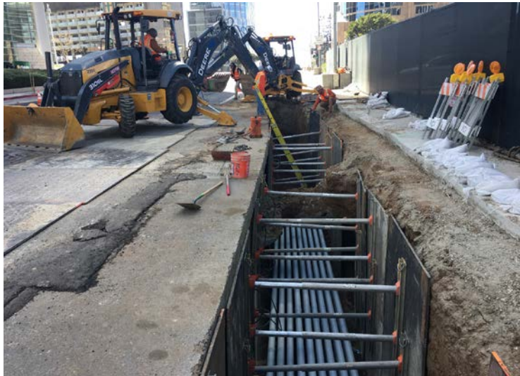
AT&T Conduit Installation in Century City
