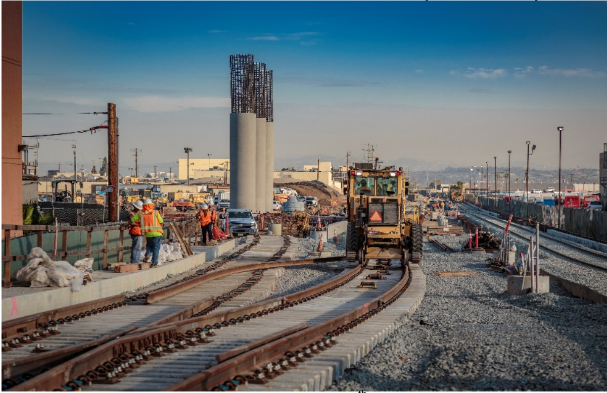
Trackwork at 96 th
