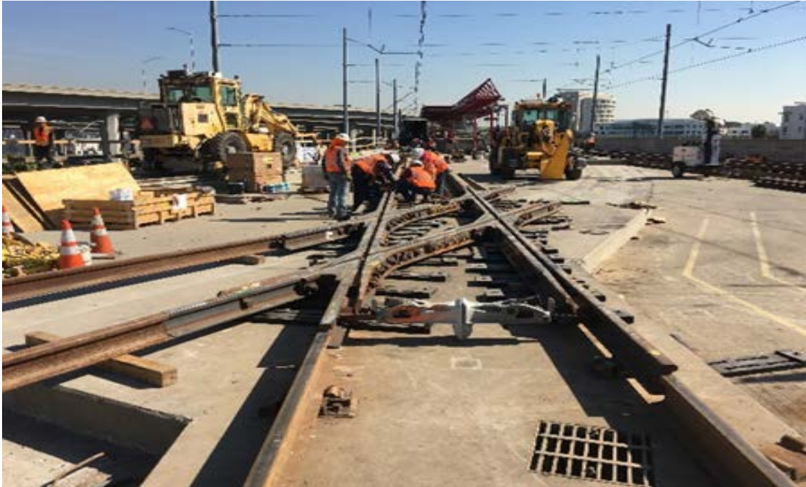
Initial set-up in progress for Green Line tie-in.
