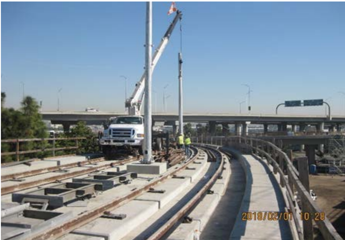
Setting overhead catenary system poles – south end.
