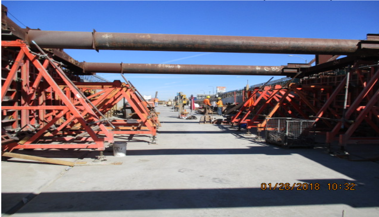
UG#3 – Removal of formwork from walls along the north U-section.
