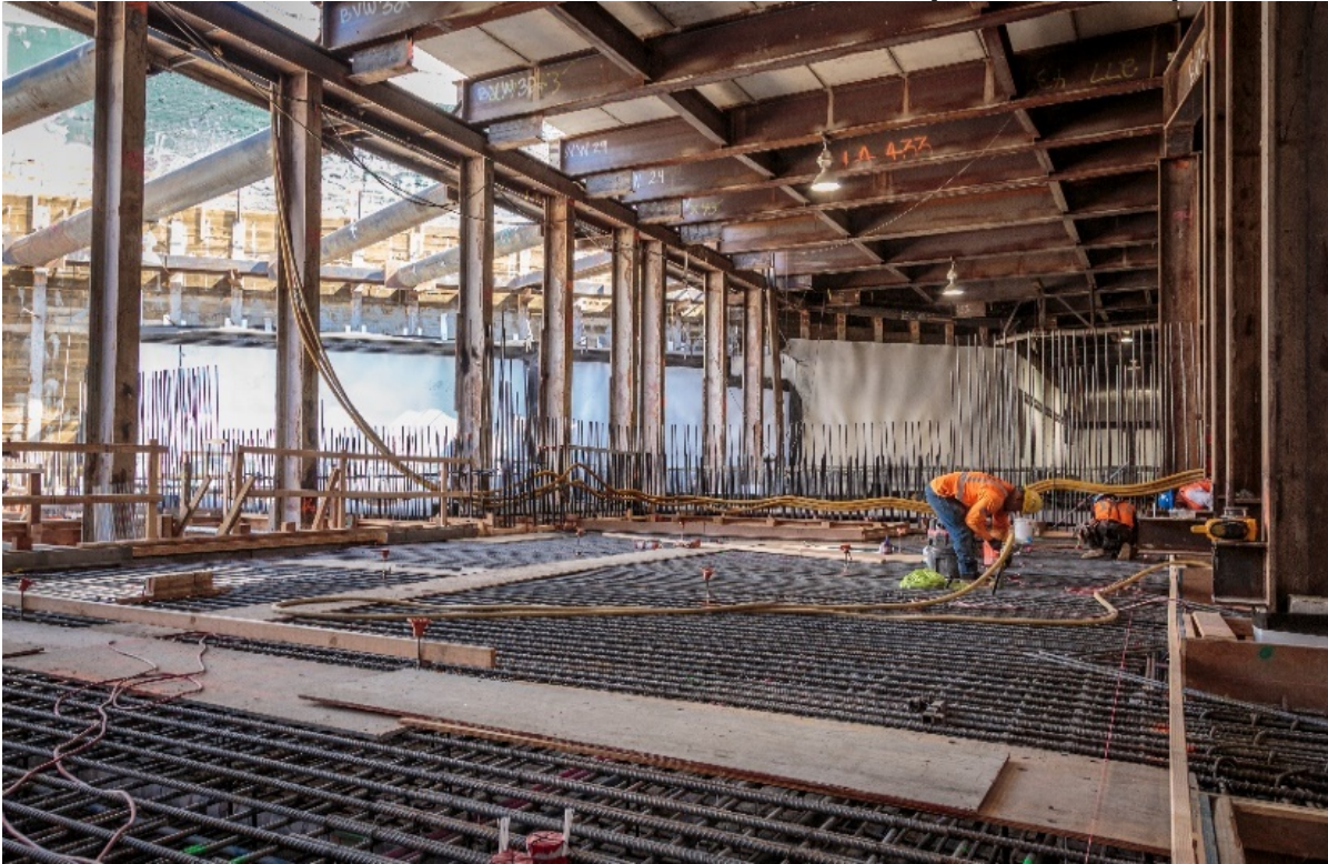
Leimert Park Station – Installing rebar for concourse concrete placement.
