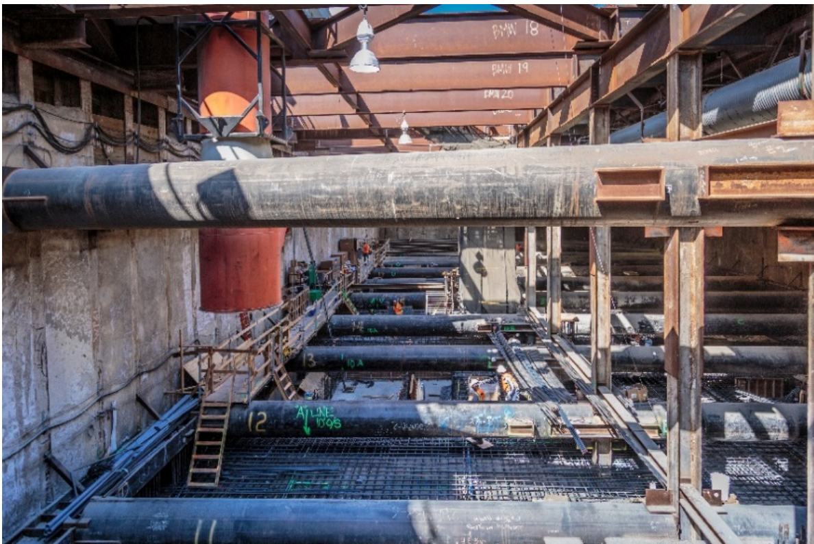
MLK Jr. Station – Installing rebar for concourse concrete placement.
