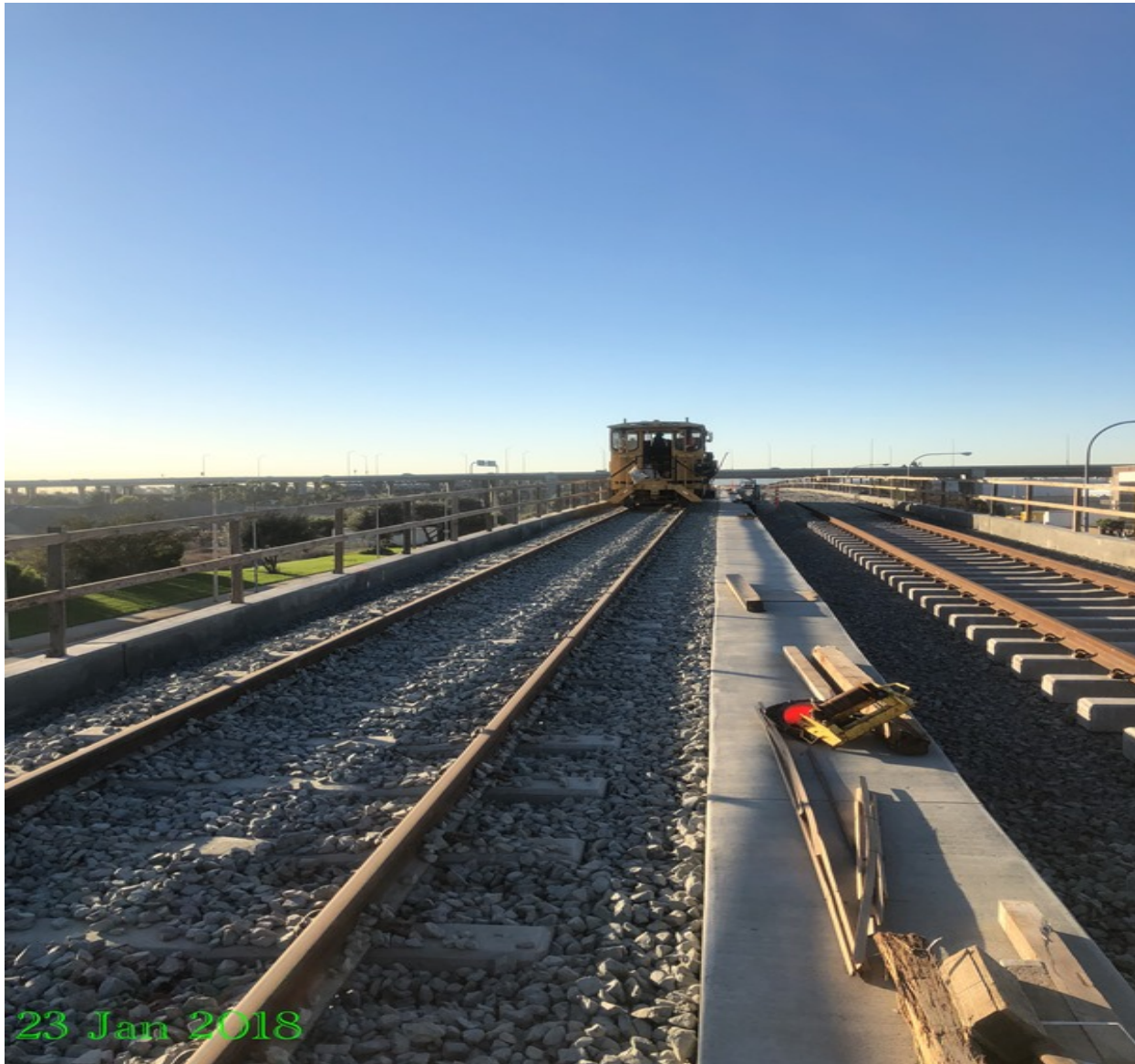
111 th Street Bridge – Tamping top ballast on track.
