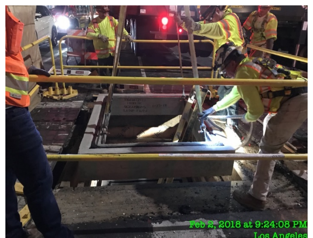
Setting manhole rings and cover at Vault 805 on Flower Street
