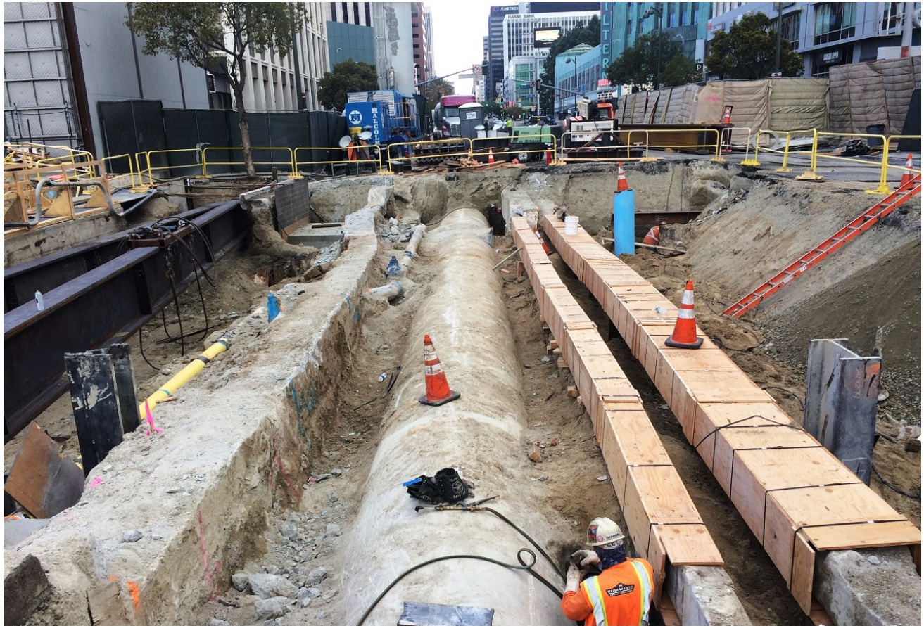
Wilshire/Western Station Street Decking Operation
