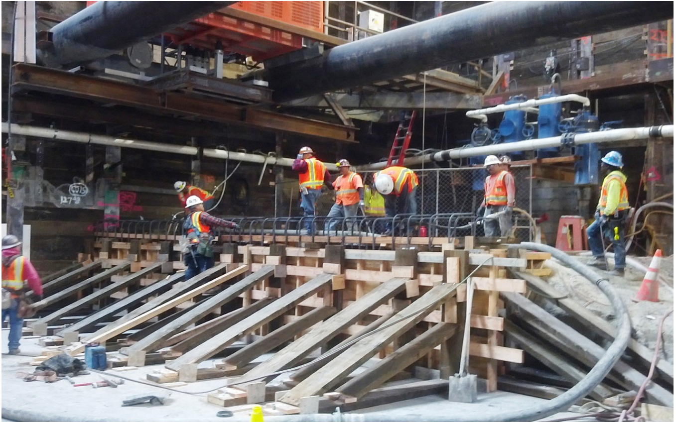
Wilshire/La Brea Station TBM Slab
