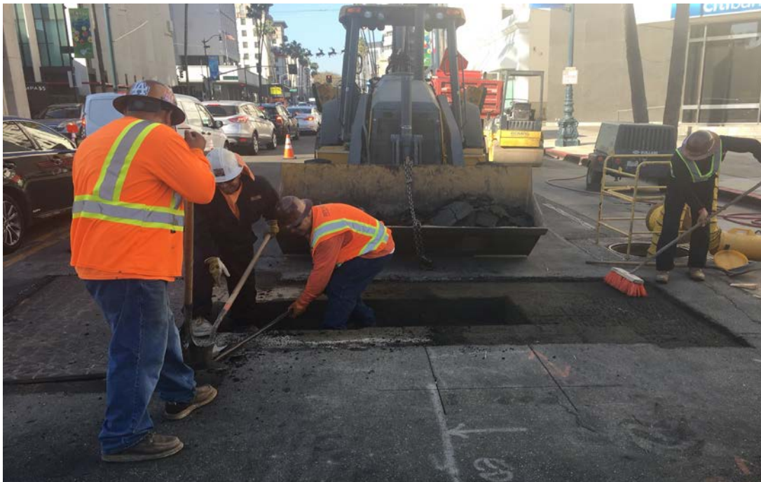
Southern California Edison (SCE) Relocation Work in Beverly Hills
