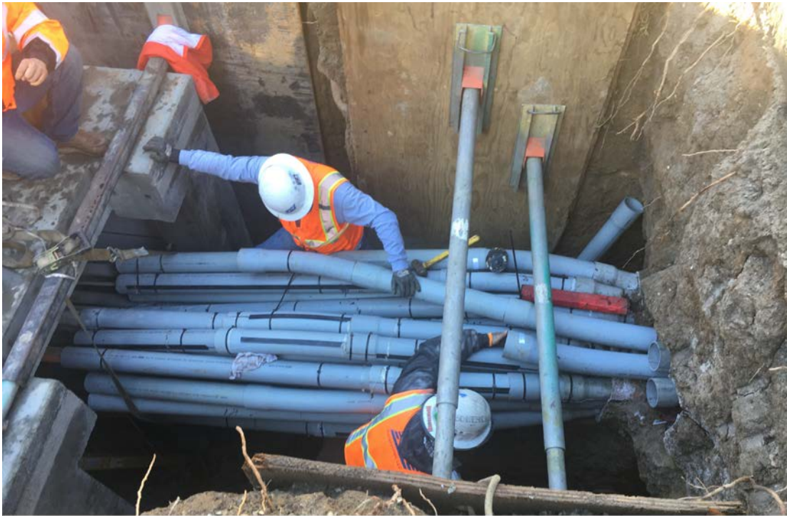
AT&T Conduit Installation in Century City
