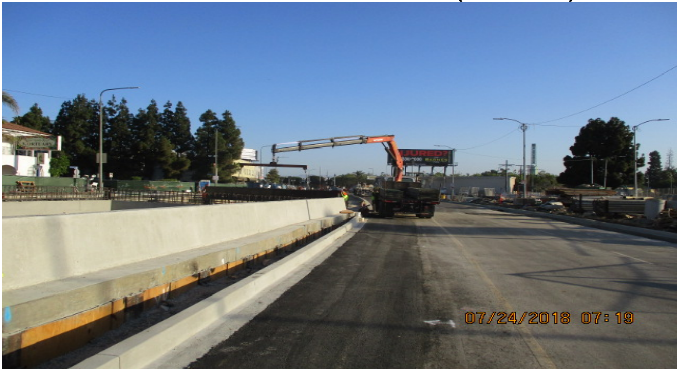
UG4 – Installation of formwork for the barrier wall.
