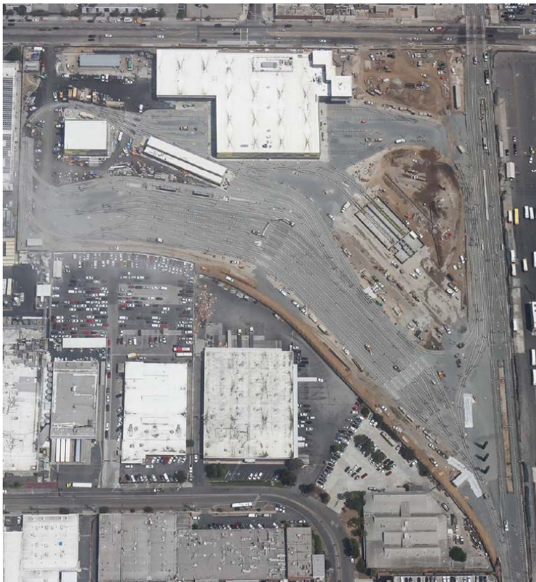
Aerial of Southwestern Yard site.
