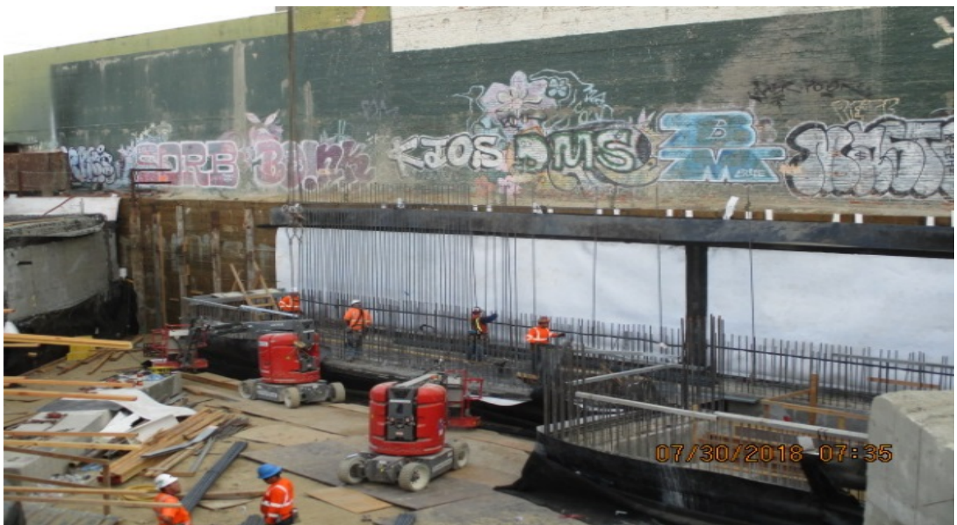
LEIMERT PARK STATION – Rebar installation at the emergency ventilation shaft.
