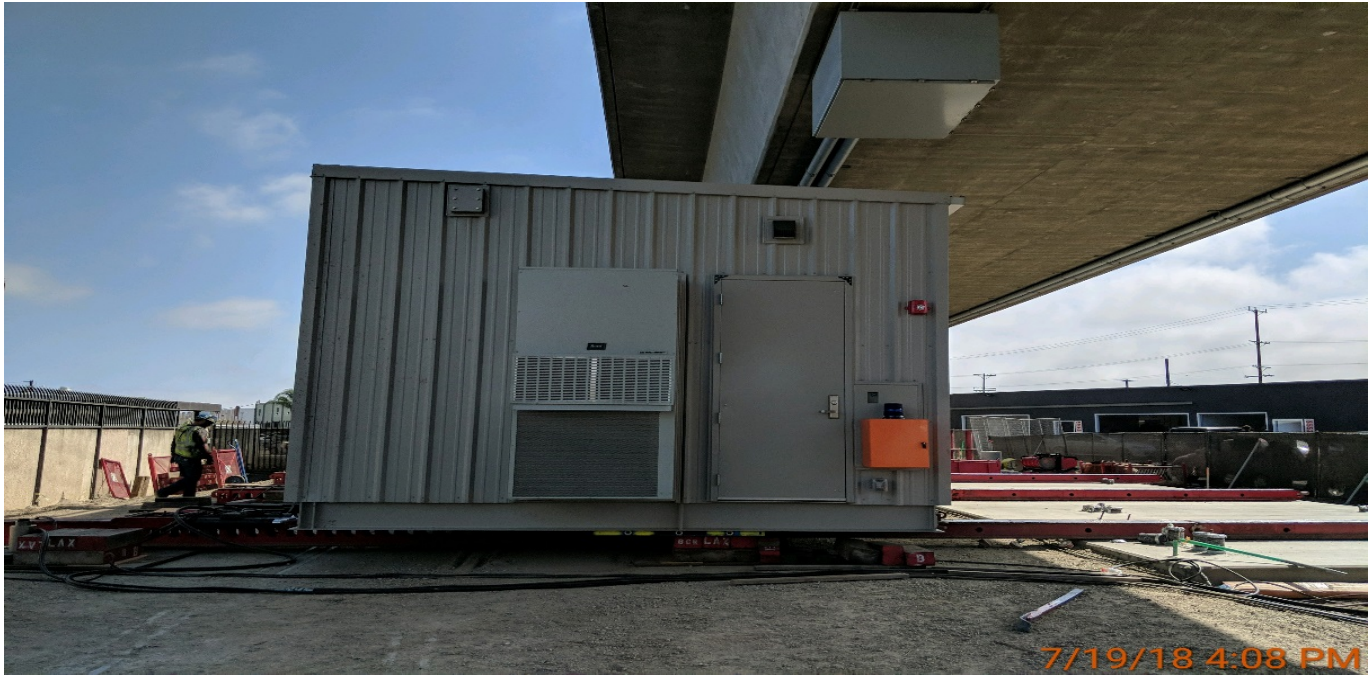
TPSS- TPSS#3 – Preparation for the Jack and Slide to Set TPSS.
