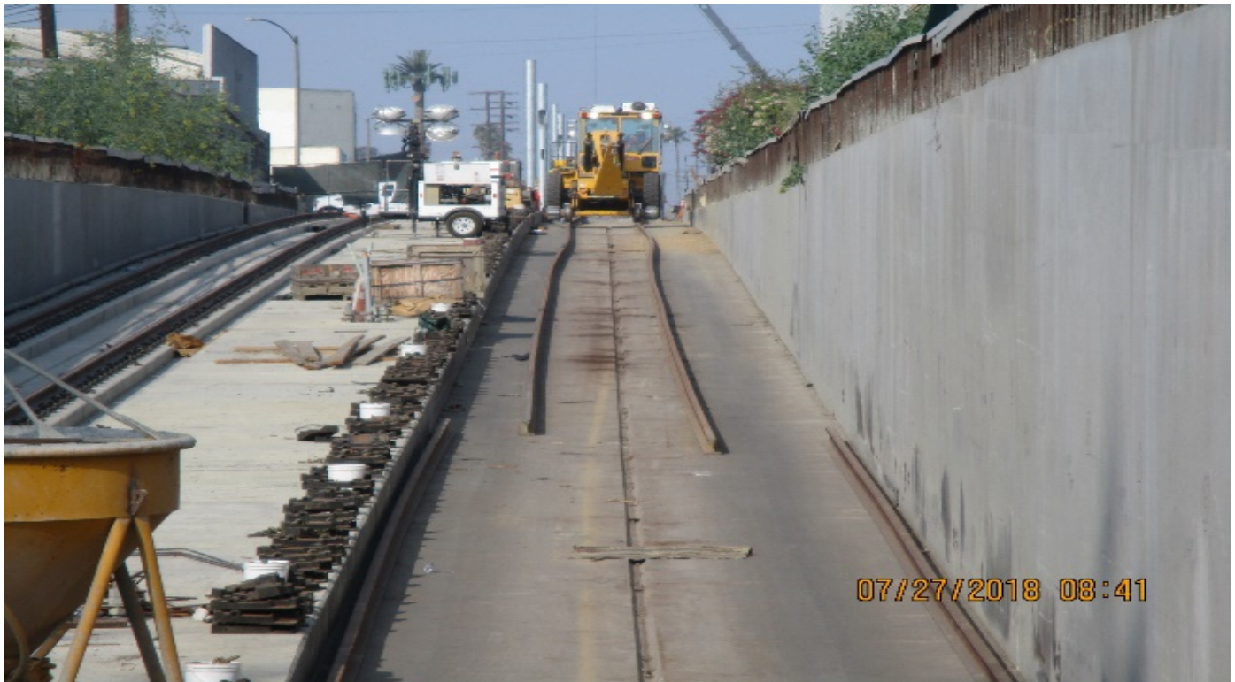
UG3 - SB track work at the south tunnel portal
