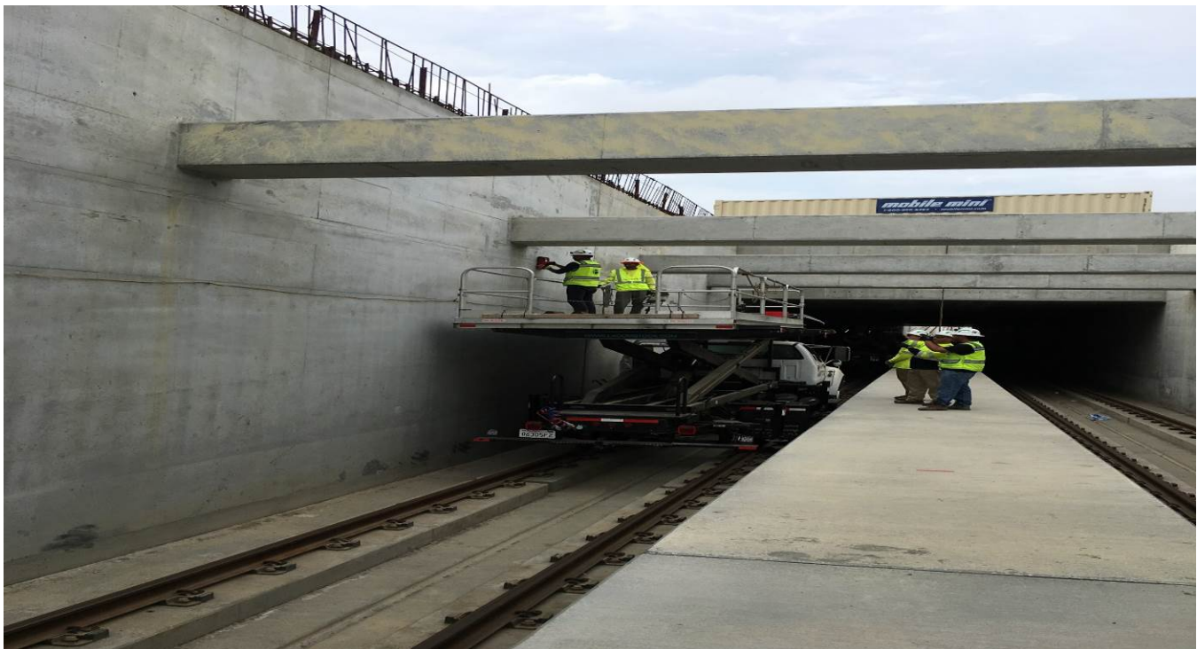
UG1 - LKC Crew Scanning for Rebar at UG-1.
