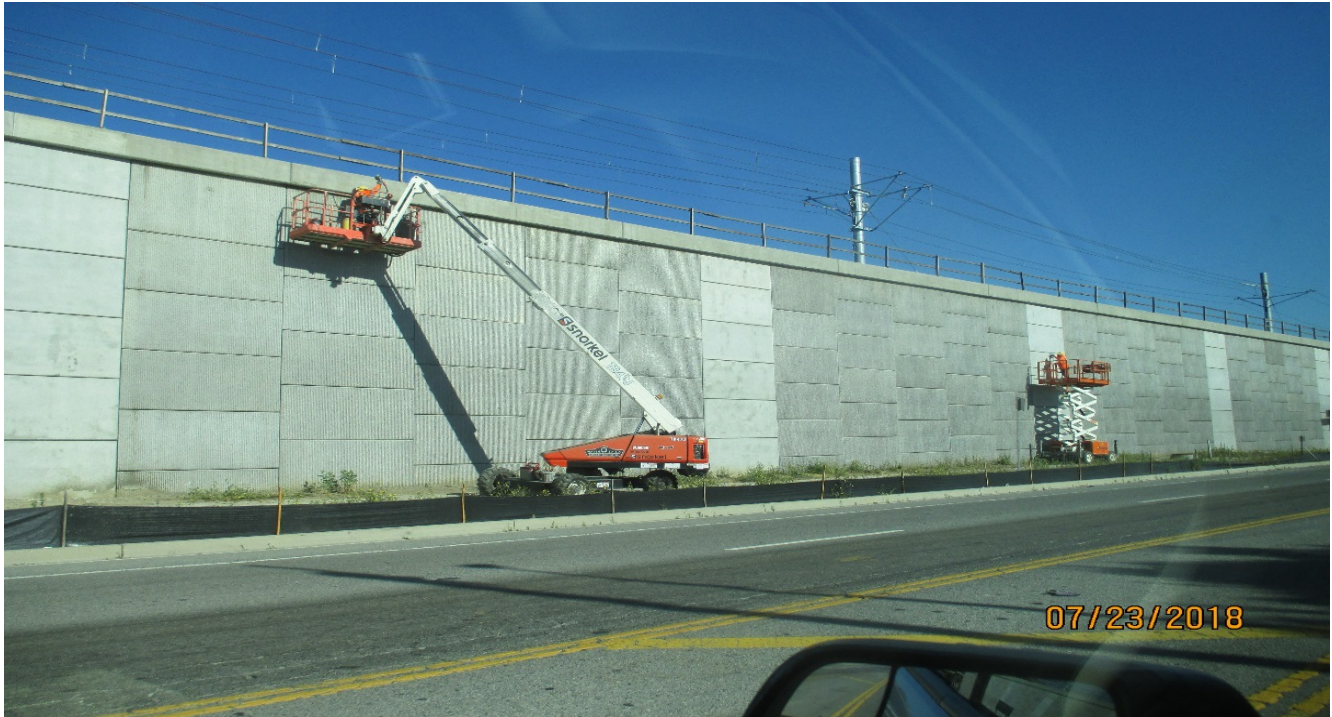
MSE 17 – Working on the Concrete Finish at MSE RW 1716+63.
