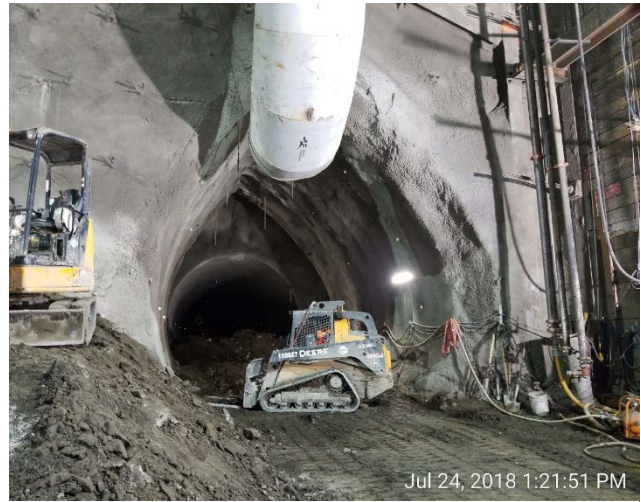
SEM right drift excavation
