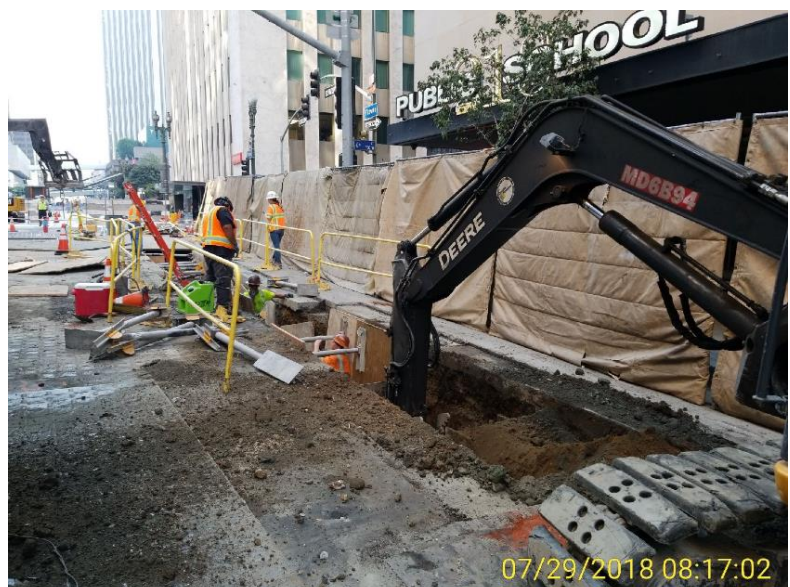
Excavation for cap beam installation on Flower Street
