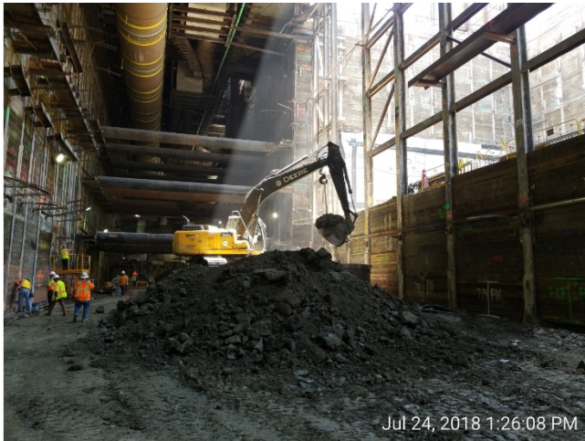
Excavation in Historic Broadway Station
