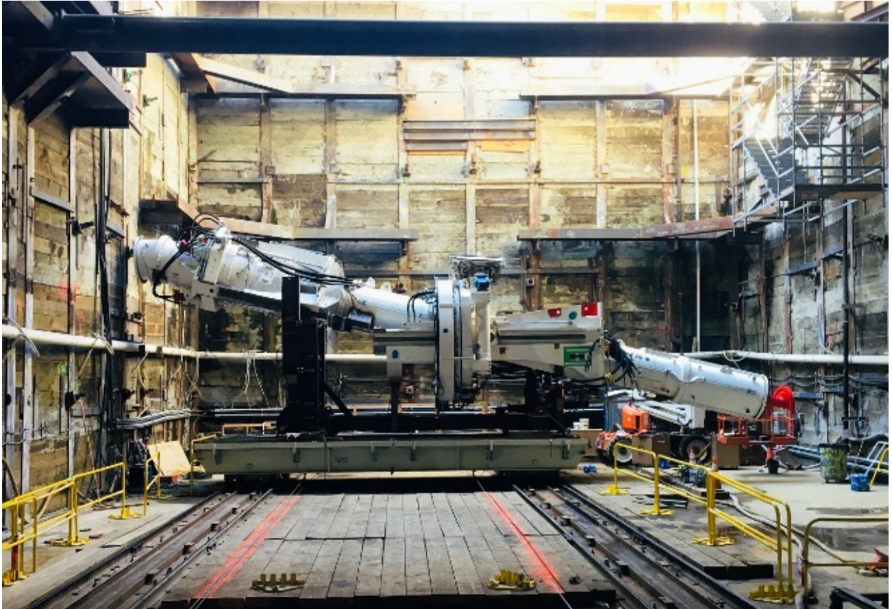
TBM Screw Conveyor at Wilshire/La Brea Station
