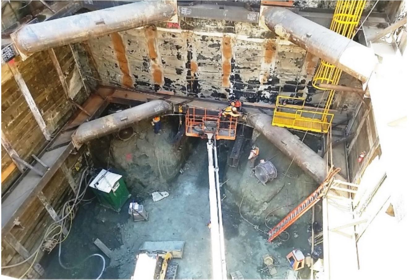
Bottom of Blast Relief Shaft at Wilshire/Western Site
