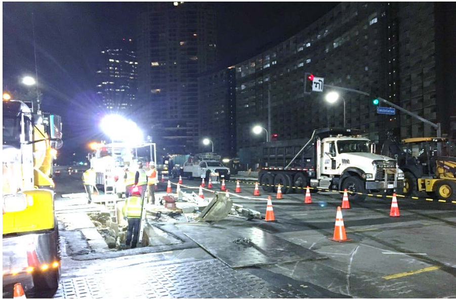
LADWP Power Utility Work in Century City
