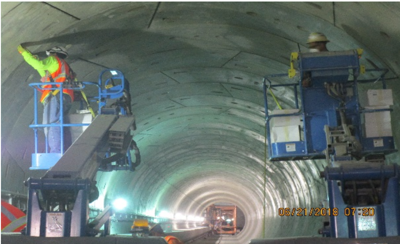
TUNNEL – Installation of the radiating cable brackets in the NB tunnel between Expo and MLK stations.
