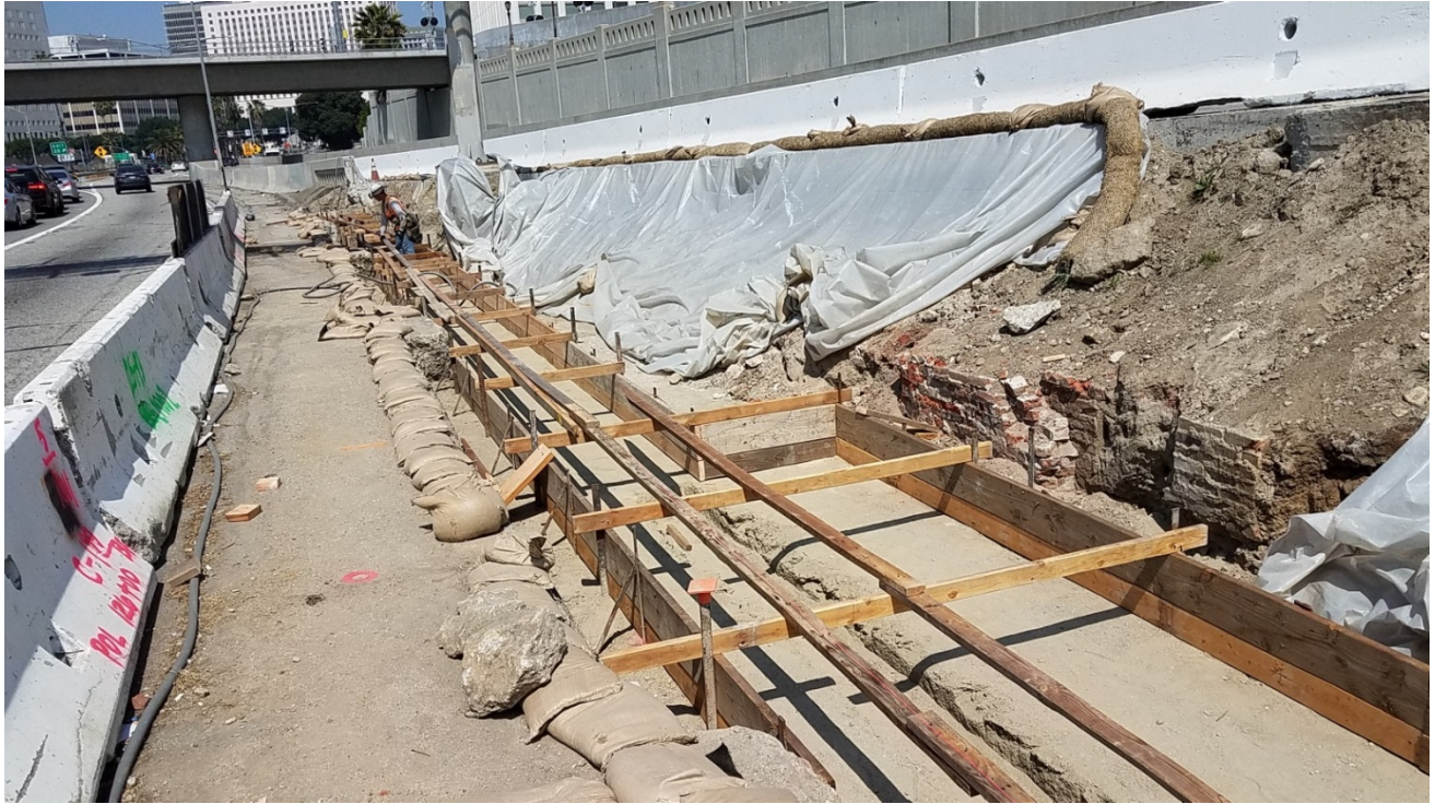
Forming retaining wall. Note bricks.
