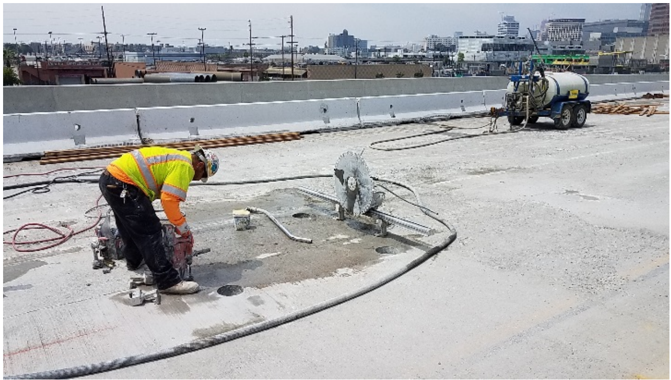
Cutting stair opening in deck.
