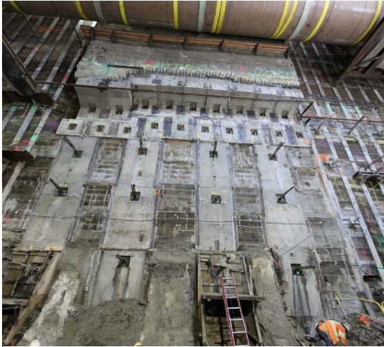
Underpinning of LA Times Building complete
