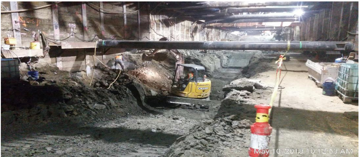
Excavation and lagging under Flower Street
