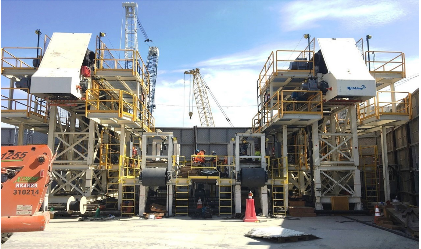
Tunneling Conveyor Assembly at Wilshire/La Brea Station
