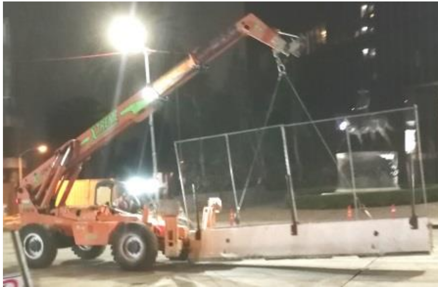
K-Rail Installation in the City of Beverly Hills
