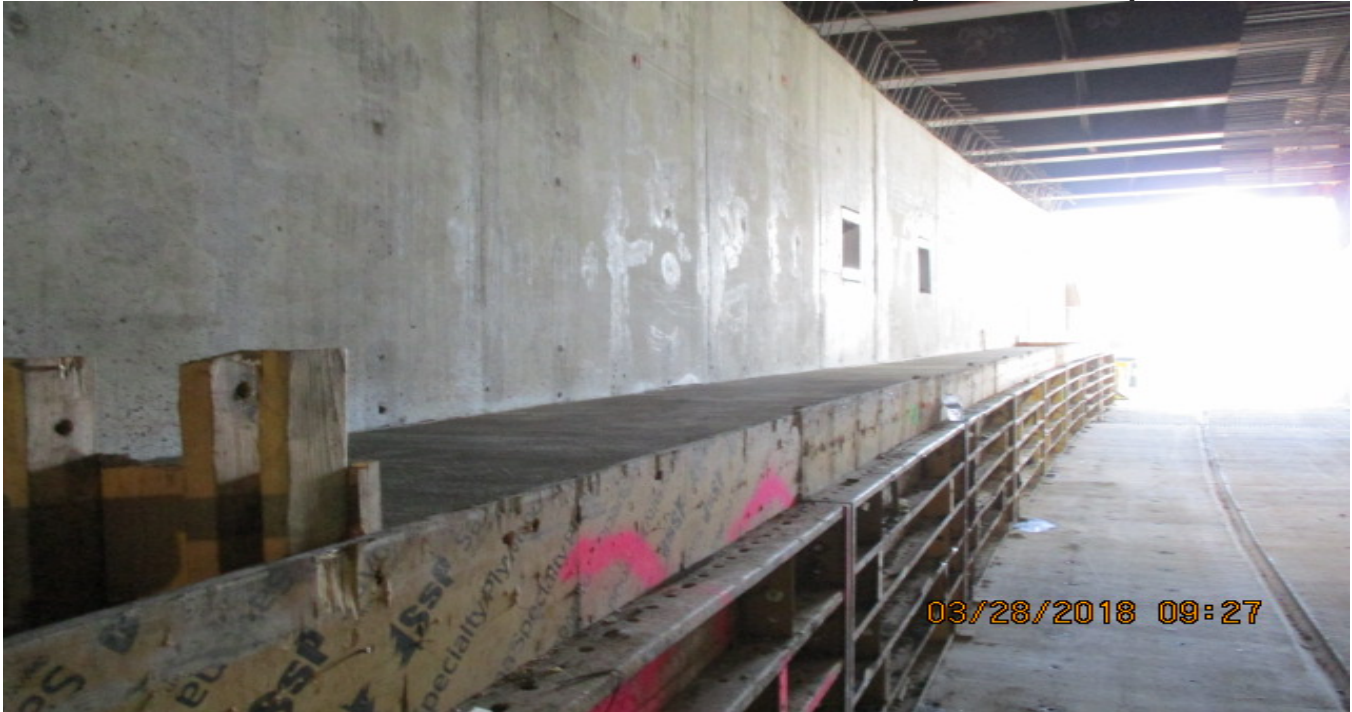
UG4 – Southbound walkway forms (pre-strip).
