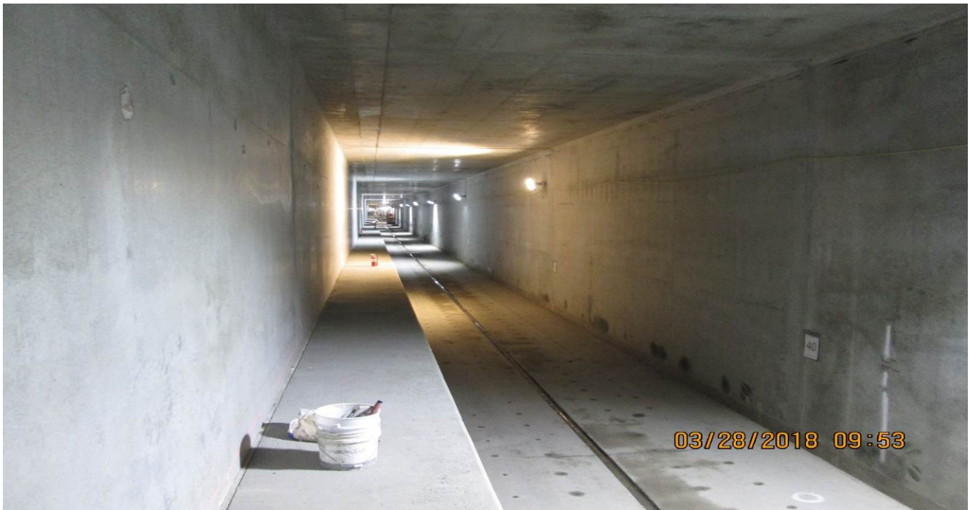
UG3 - Southbound tunnel with completed emergency walkway.
