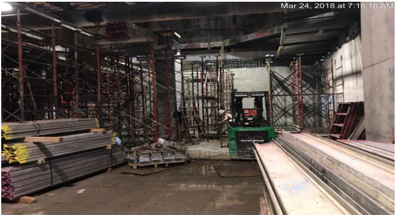
MARTIN LUTHER KING JR. STATION Installation of false work for phase 2 roof construction.
