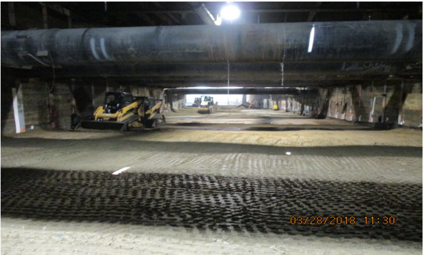
UG4 – Grading and compaction of backfill at roof level.
