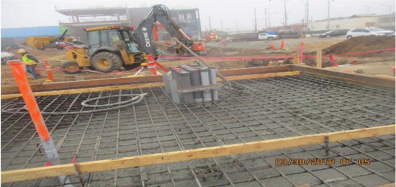
TPSS - TPSS 4- Placing concrete for slab on grade.
