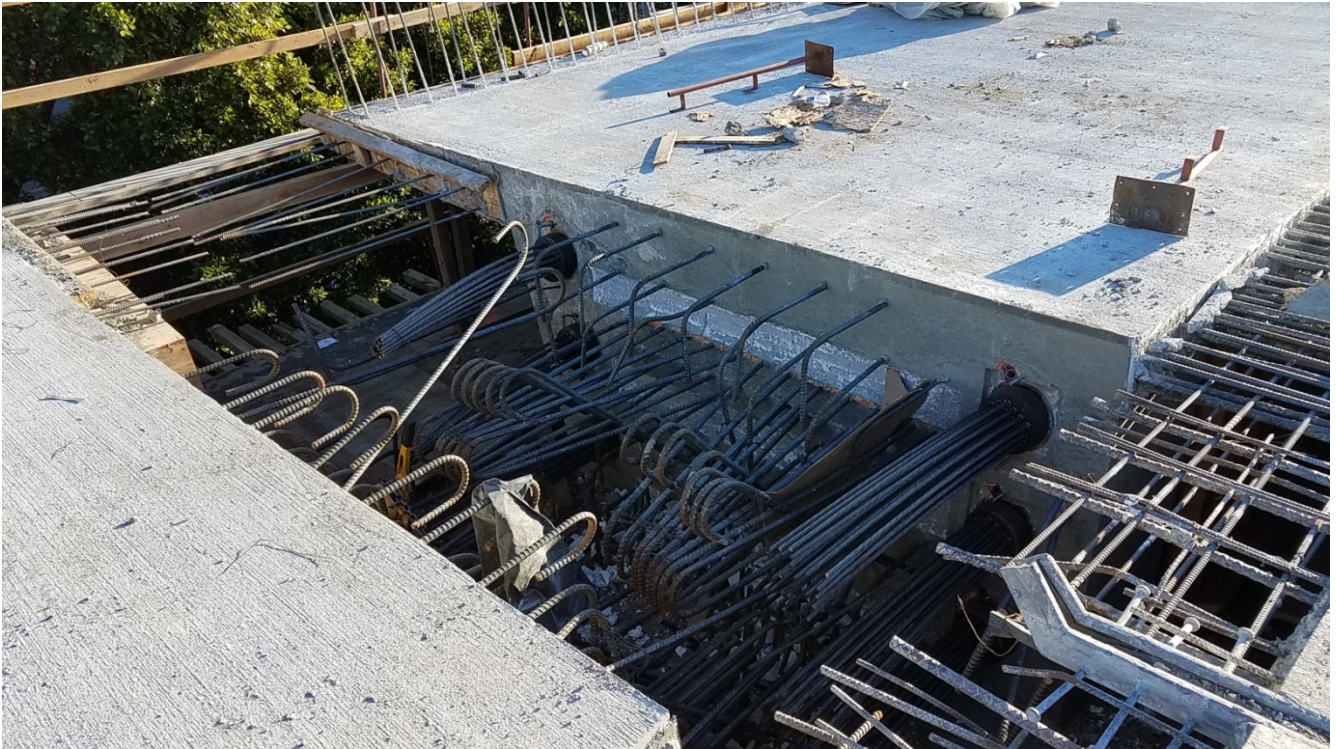
Post Tensioning Frame 4 Left.
