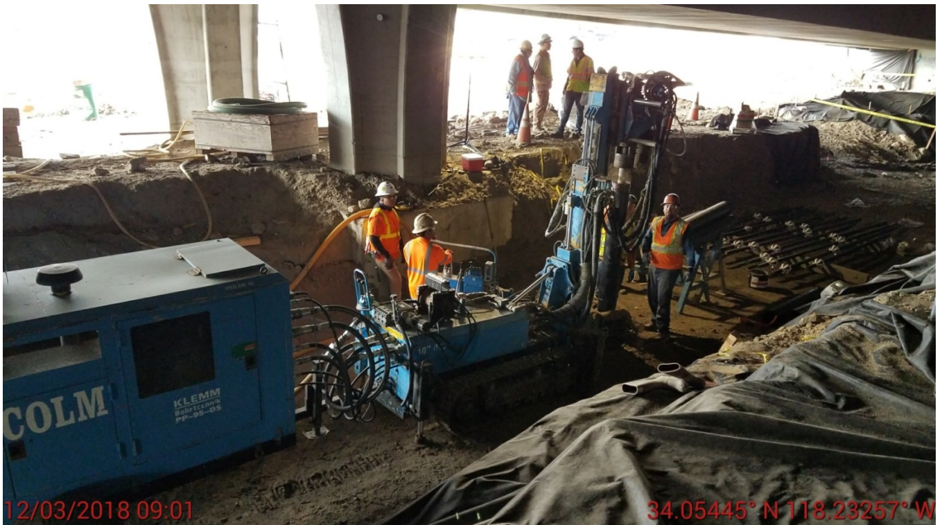
Drill for Micropile Test.
