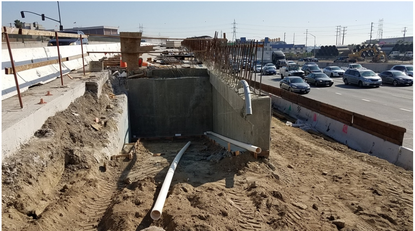
Drain at Abutment 1.
