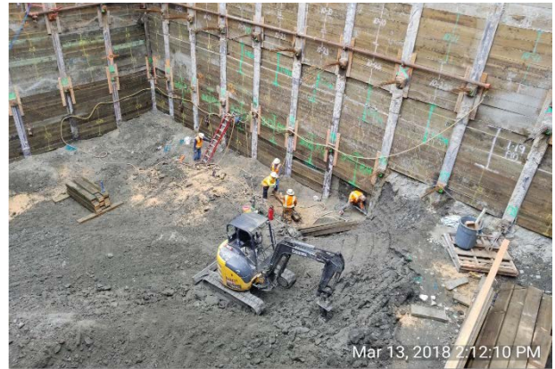
Excavation, lagging and tieback installation at Historic Broadway Station
