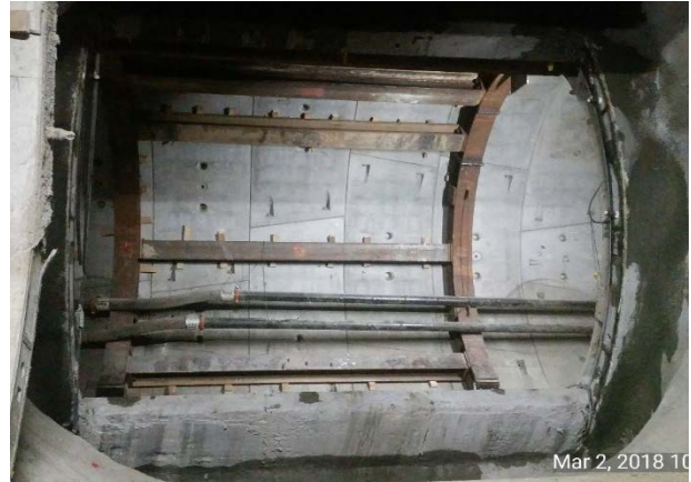
Cross Passage #3 breakthrough
