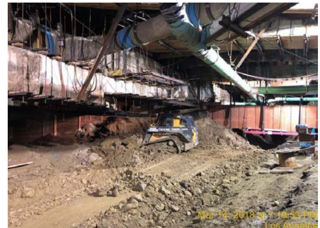
Utility support and excavation beneath Flower Street
