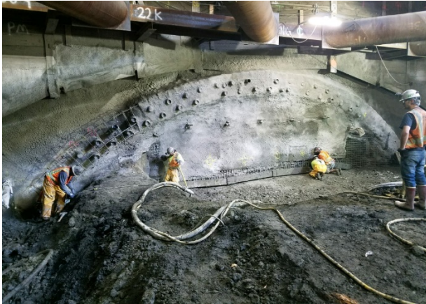
SEM canopy pipe installation
