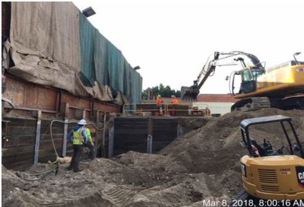
Excavation and utility support resuming at Alameda and 1st Street intersection
