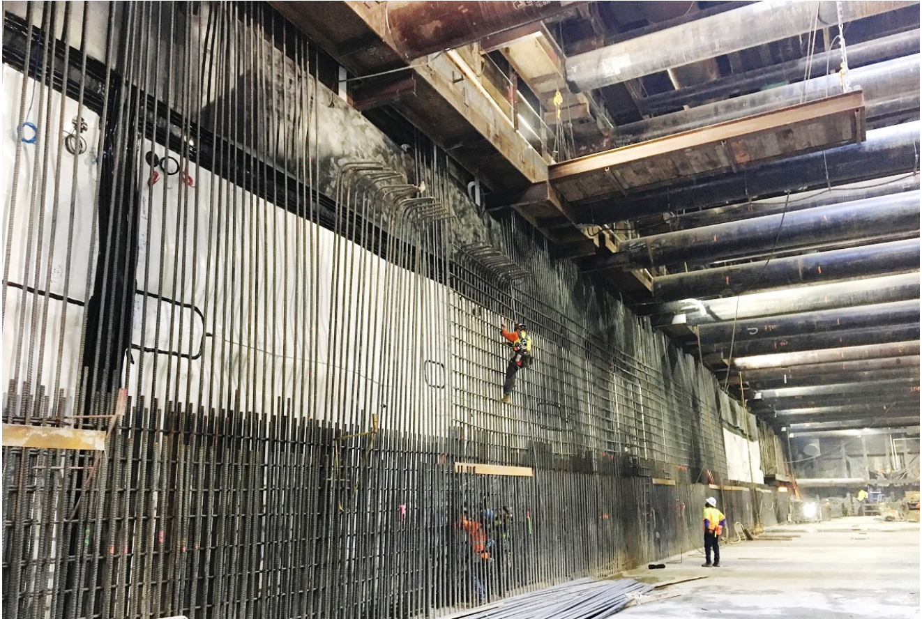
Wilshire/La Brea Station
