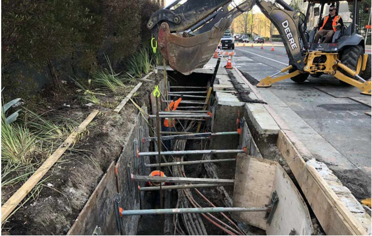
AT&T Utility Work in Century City
