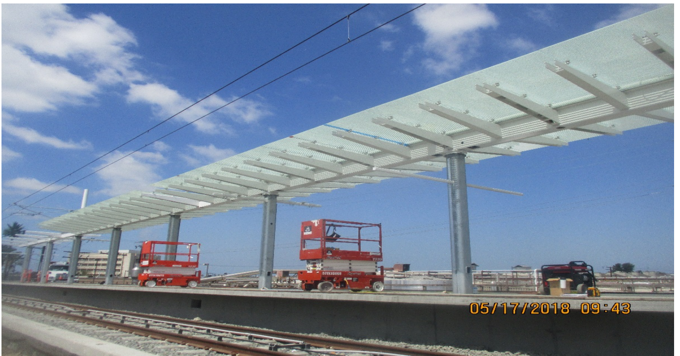
LA BREA AT- GRADE STATION - caulking placement on glass panels.
