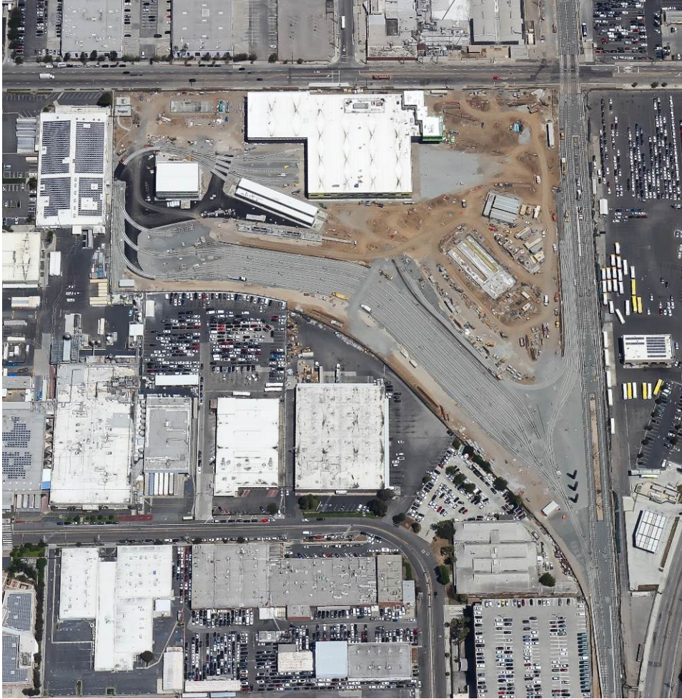
Aerial view of Southwestern Yard.
