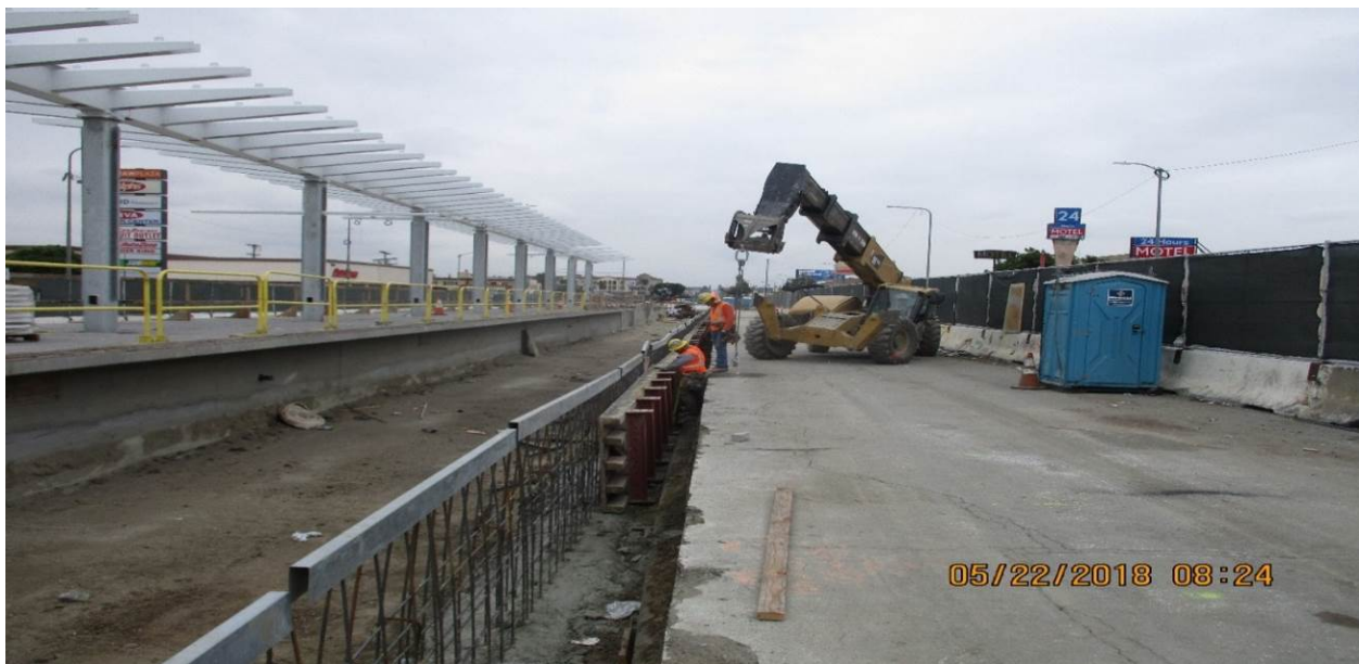
HYDE PARK STATION - Installation of formwork for the south ballast wall.
