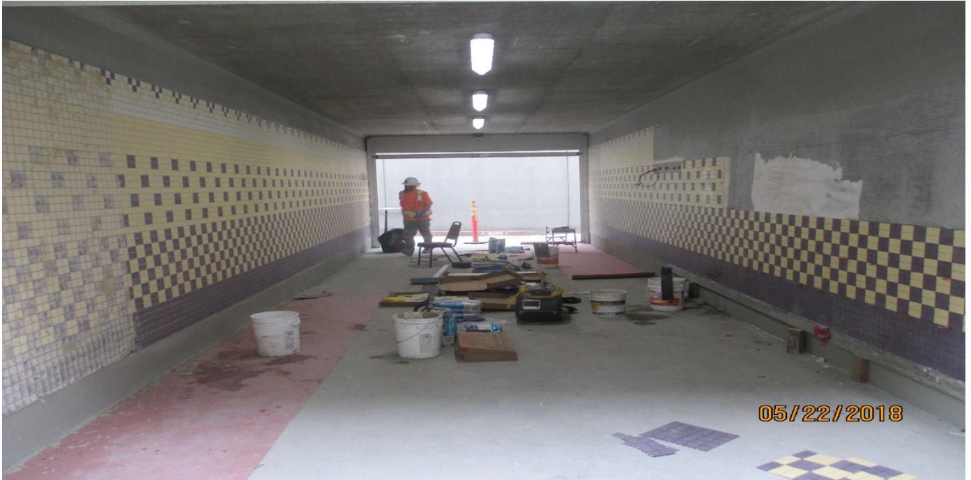
FCBC - setting tile for the walkway underpass.
