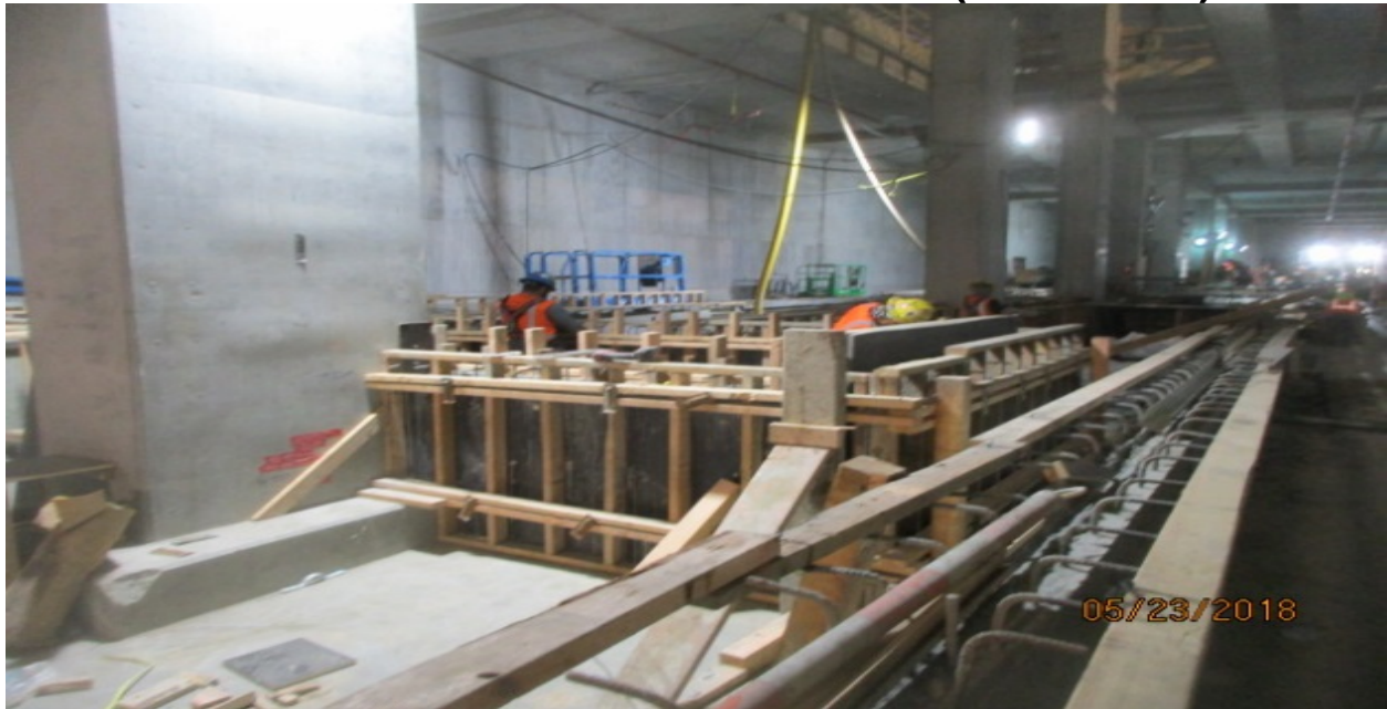
LEIMERT PARK STATION - installation of formwork for platform walls.
