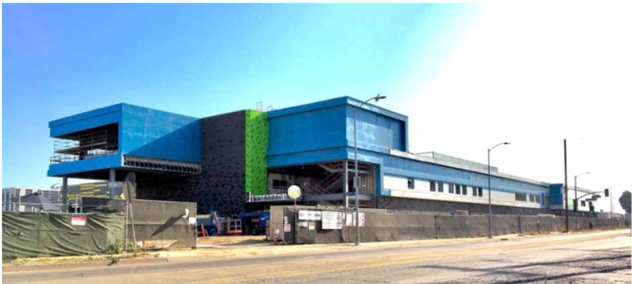
Main shop within the Southwestern Yard site.
