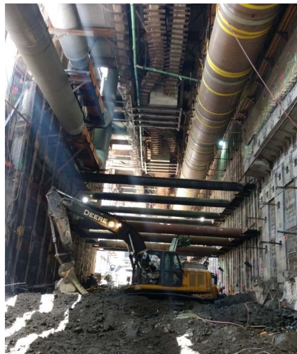
Excavation in ancillary area at Historic Broadway Station
