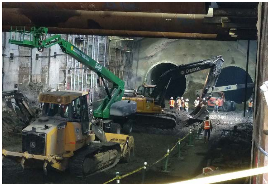
Sequential Excavation Method (SEM) underway at Historic Broadway Station
