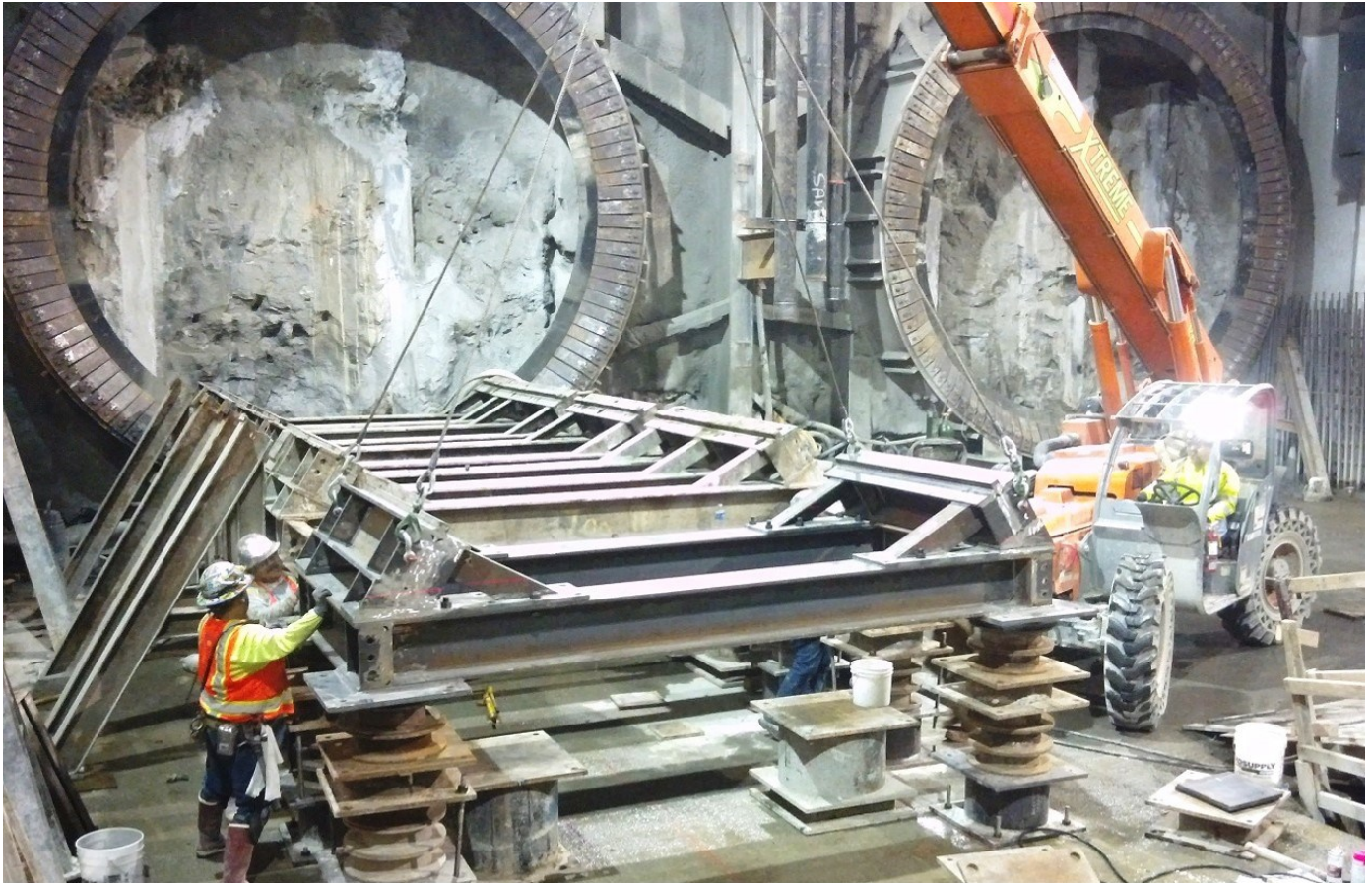
TBM Cradle at Wilshire/La Brea Station
