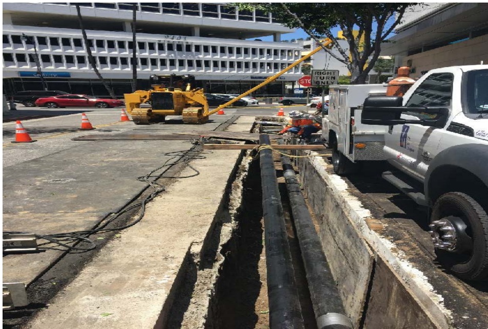
SCG Utility Work in Beverly Hills
