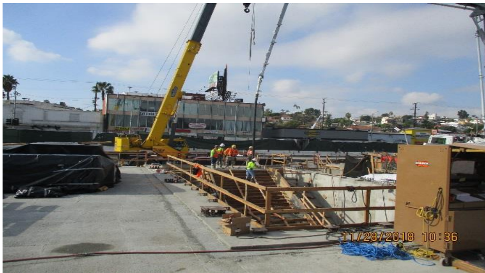
Concrete placement for Stair #1 at Leimert Park Station entrance structure
