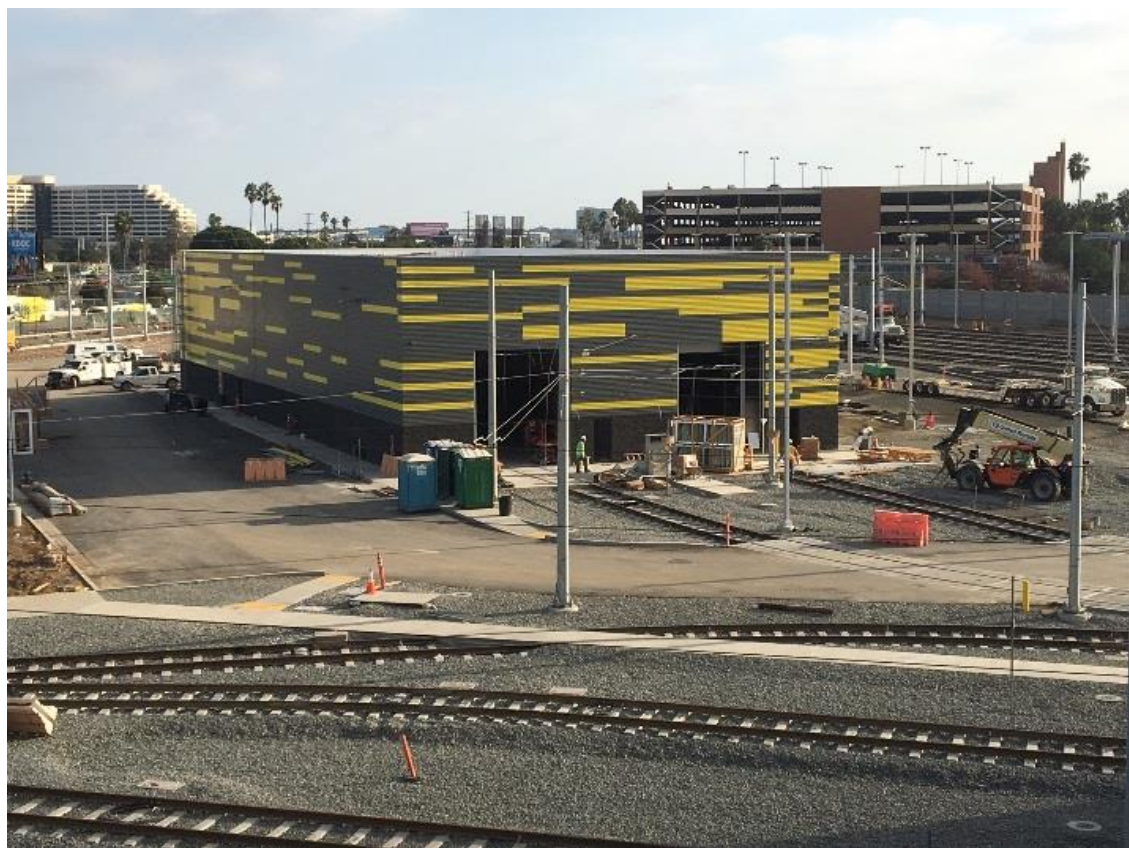
Looking southeast at Paint and Body Shop in Southwestern Yard
