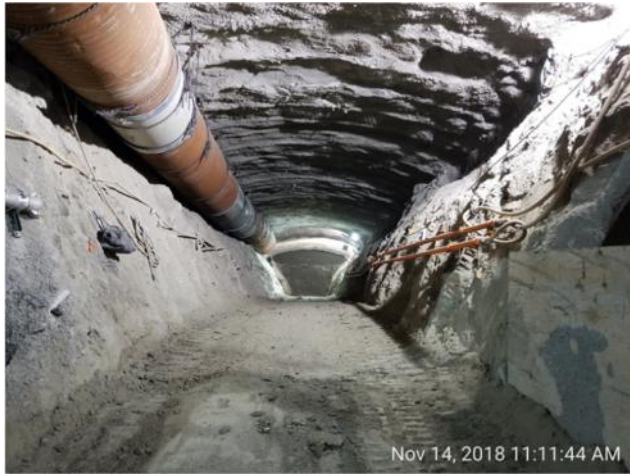
SEM Cavern center top drift progress
