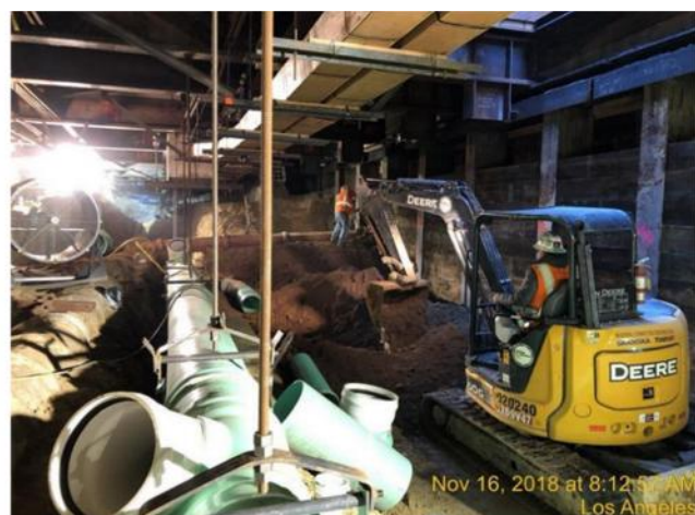
Preparations for sewer bypass under Flower St
