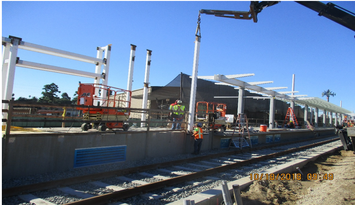
Erecting the east ticket fare gate at the West Station.
