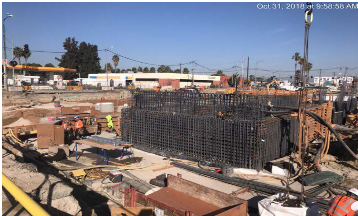
Installation of rebar for plaza level wall at Exposition/Crenshaw Station.
