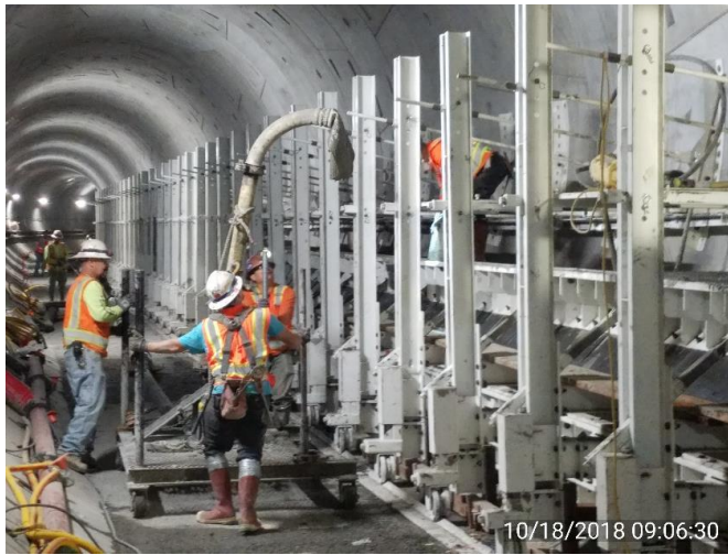
Concrete placement for Left Tunnel Walkway, Flower to Hope
