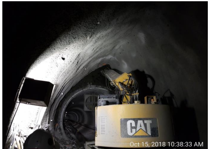
Left drift end wall excavation in SEM Cavern
