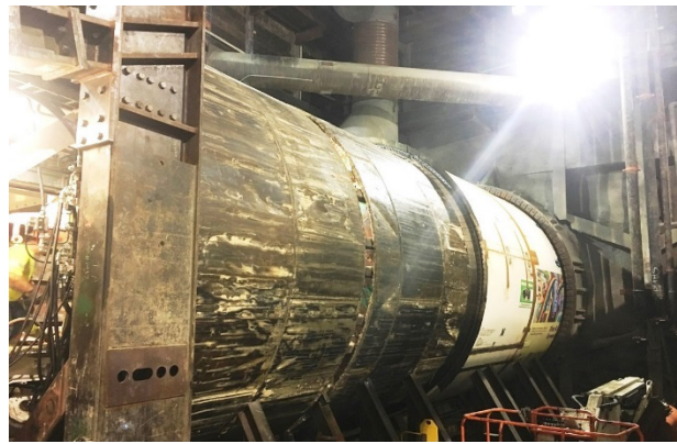
TBM Launch at Wilshire/La Brea Station
