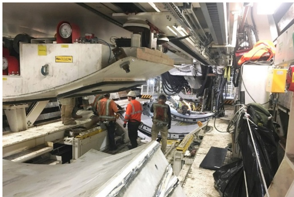
Tunnel Ring Assembly at Wilshire/La Brea Station
