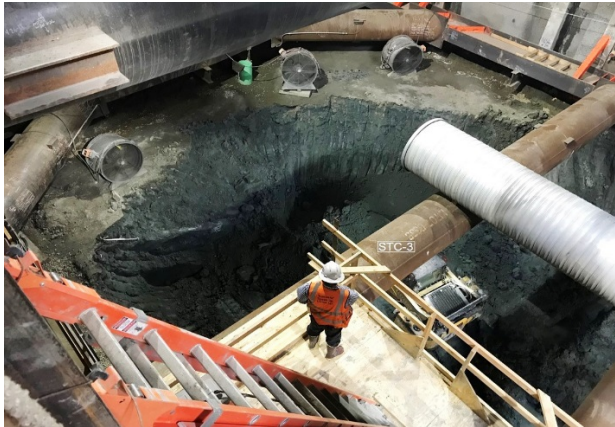
Excavation at Wilshire/Western
