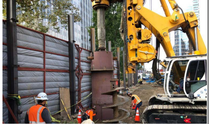
Steel Casing Installation during Test Drilling on Constellation Boulevard
