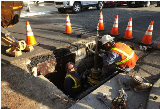
Southern California Gas Relocating Eight-Inch Gas Line in Beverly Hills
