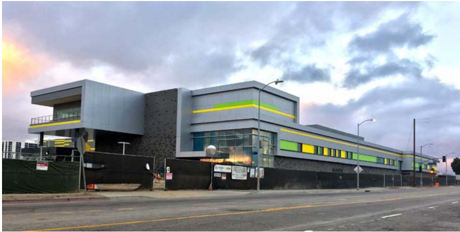
Southwestern Yard - main shop building looking southwest.
