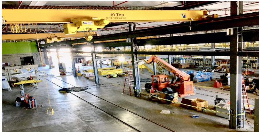
Southwestern Yard – maintenance area.
