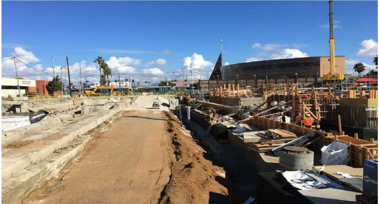
Crenshaw Blvd restoration & Expo/Crenshaw Station entrance construction near Expo Line.
