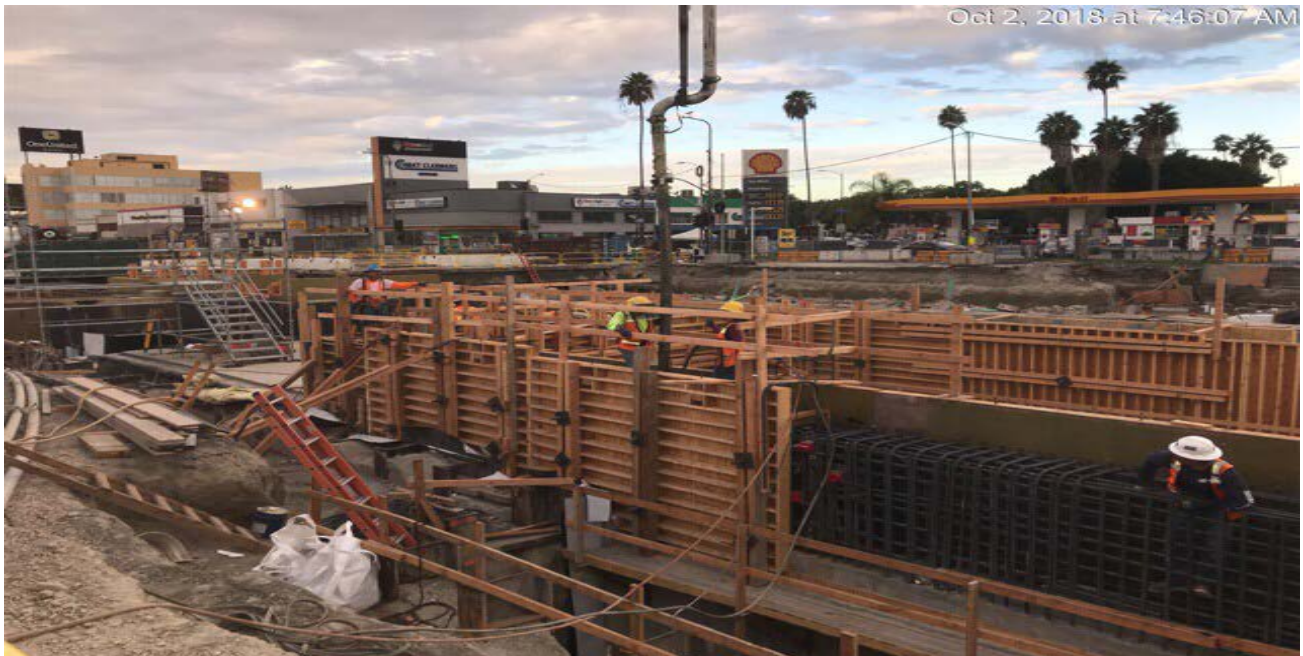
Concrete placement for wall at the plaza level Exposition/Crenshaw Station.
