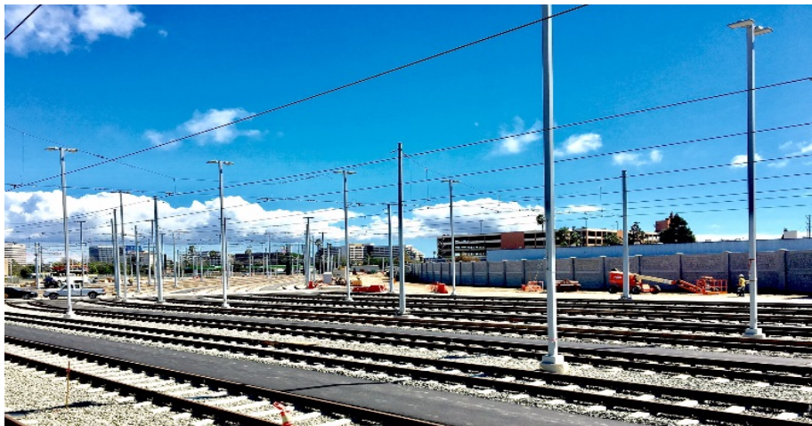
Southwestern Yard – storage tracks.
