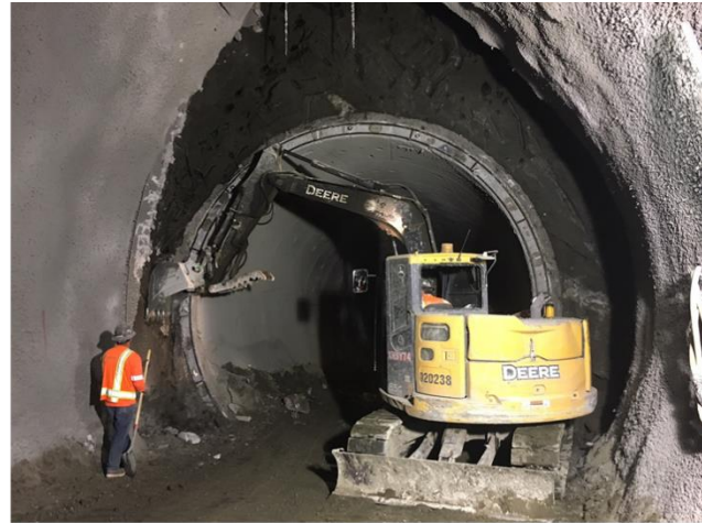
Excavation for arch on Right Drift of the SEM Cavern
