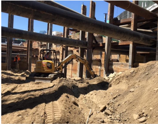
Excavation at Central
