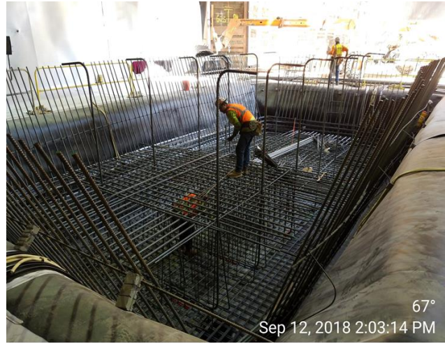
Installation of bottom mat reinforcement at west sump Historic Broadway Station
