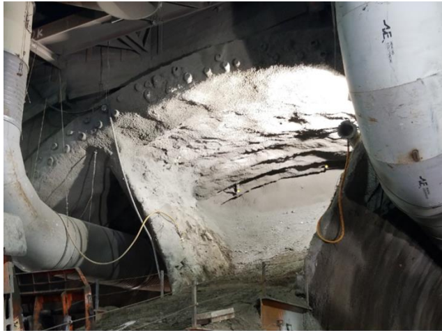
Excavation and shotcrete application at Center Drift of the SEM Cavern
