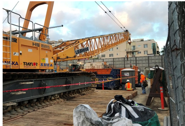
Crane at Wilshire/La Cienega Station
