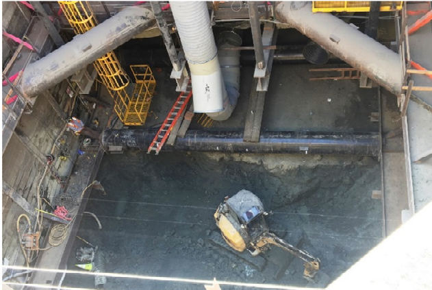
Excavation at Wilshire/Western
