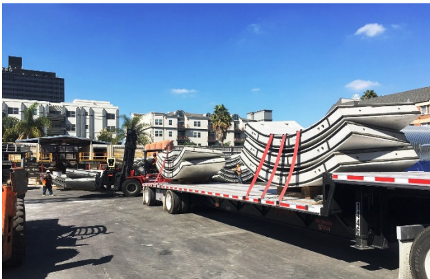
Tunnel Segments at Wilshire/La Brea Station
