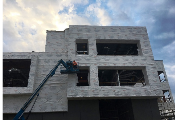
Division 20 Building – West Exterior Wall
