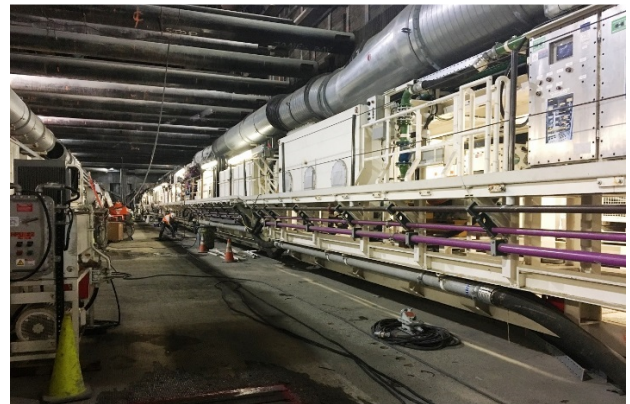
TBM at Wilshire/La Brea Station
