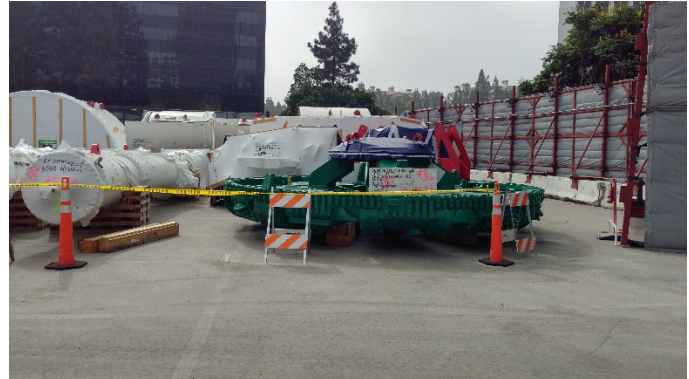
Tunnel Boring Machine (TBM) Delivery
