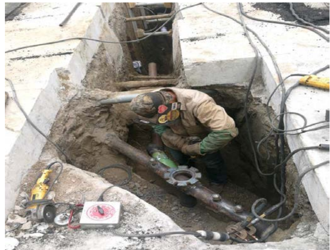
SCG Pipe Placement in Beverly Hills
