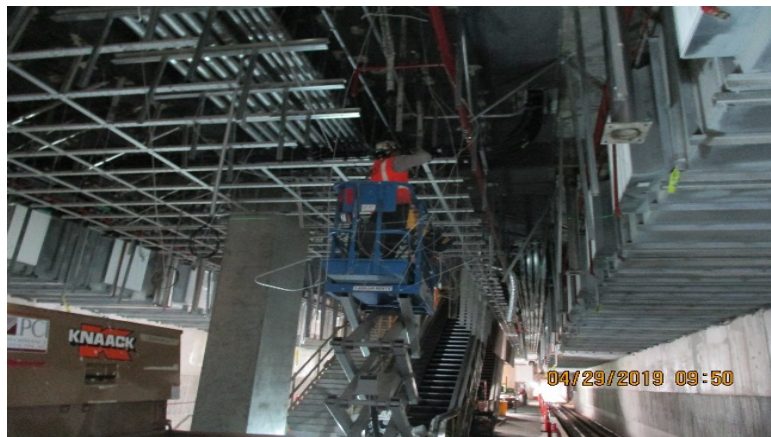
Installation of metal ceiling grid at the Leimert Park Station platform.
