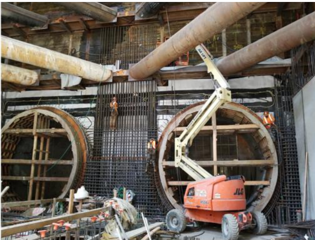
Westheadwall rebar installation at Historic Broadway Station
