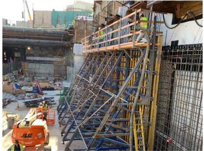
Ancillary exterior concrete wall placement at future Little Tokyo/Arts District Station
