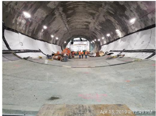
HDPE installation in SEM Cavern
