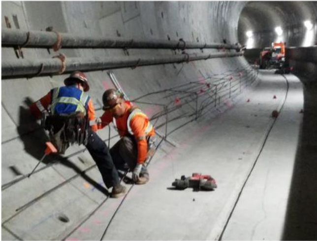
Floating Slab Track curb rebar installation
