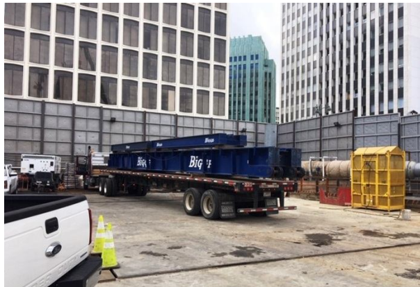
Delivery of Gantry Crane at Wilshire/Western
