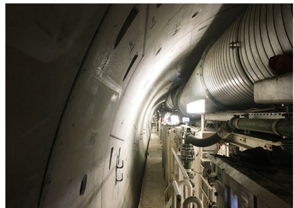
View of Reach 1 Tunnel Lining
