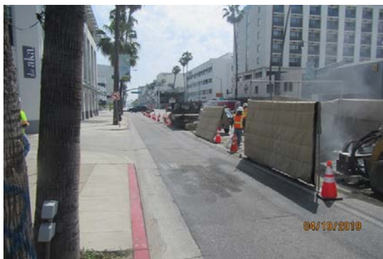
Utility Potholing Activities in Beverly Hills
