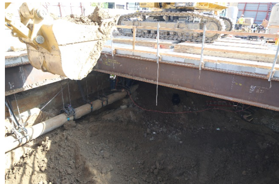
Utility Supported in Place in Century City
