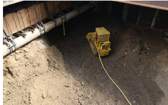
TBM Launch Box Excavation in Century City
