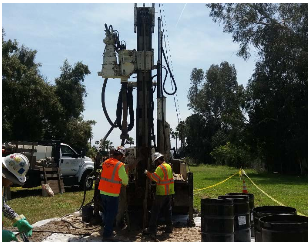
Geotechnical Boreholes at VA for Tailtrack Exit Shaft
