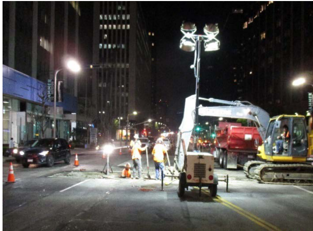
LADWP Water Relocations
