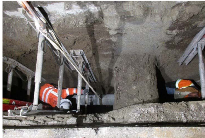
LADWP Water Fire Service Relocation
