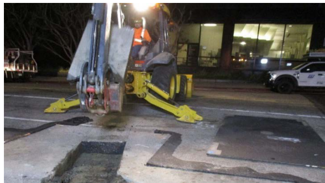
Joint Trench Excavation and Potholing
