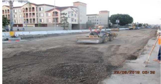
UG STRUCTURE #3 – Continued backfill and compaction between 60 th and 63 rd Street.
