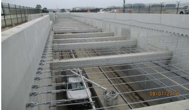
UG STRUCTURE #1 – Continued barrier installation.
