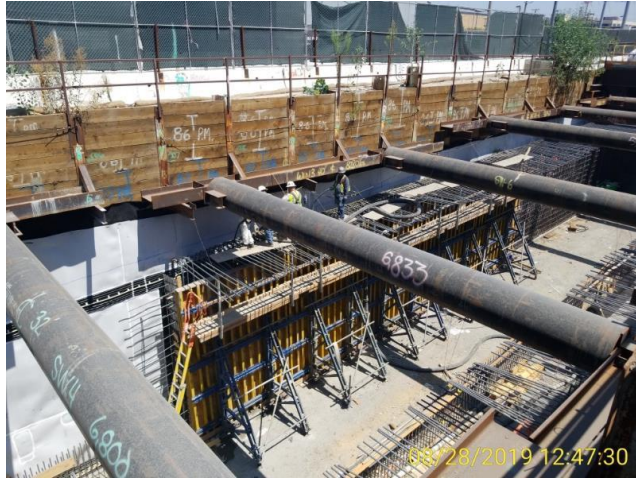
1st Street Cut/Cover Walls Pour Prep
