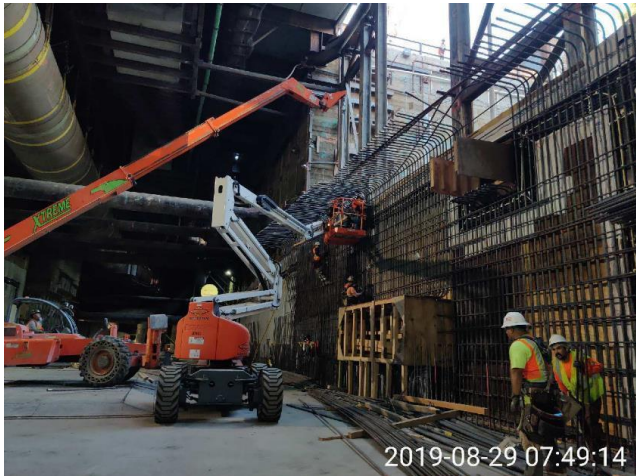
Rebar installation at Wall D 2nd lift at Historic Broadway Station
