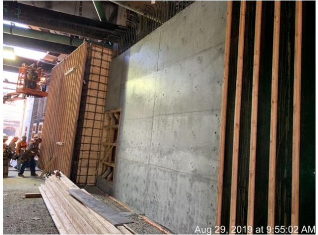
1st/Alameda Wye Formwork/Rebar Installation
