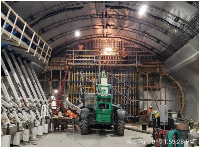
Rebar placement of Headwall in SEM Cavern
