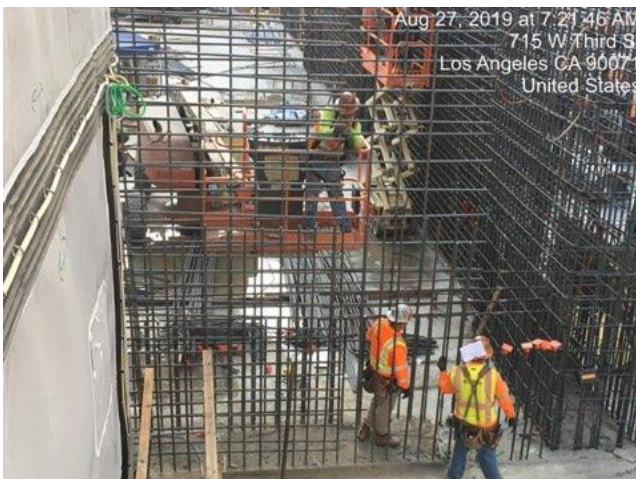
Rebar installation at Ancillary Wall of Grand Av Arts/Bunker Hill Station
