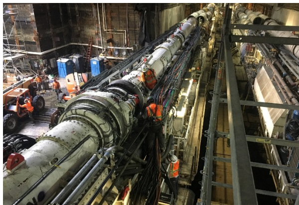
TBM Assembly at Wilshire/La Brea Station
