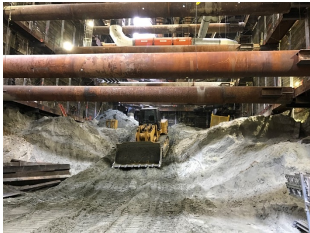
TBM Launch Box Excavation in Century City
