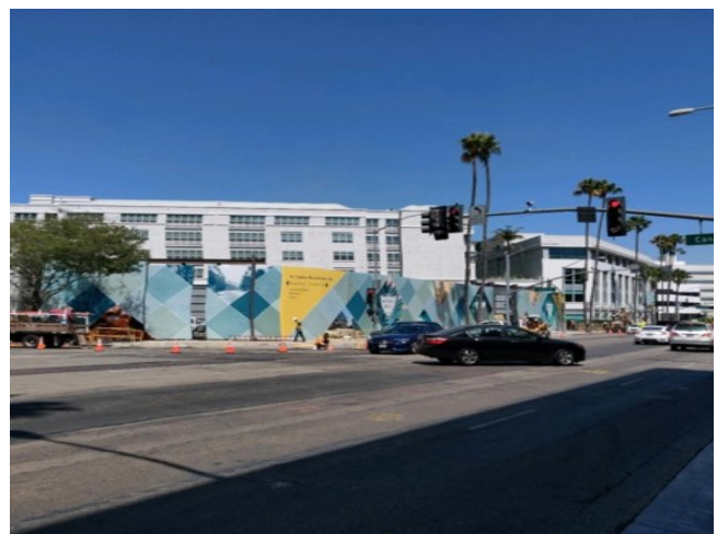
Canon Staging Yard Sound Wall Installation in Beverly Hills
