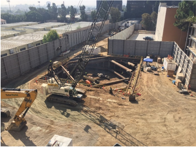
Tunnel Access Shaft Excavation in Century City
