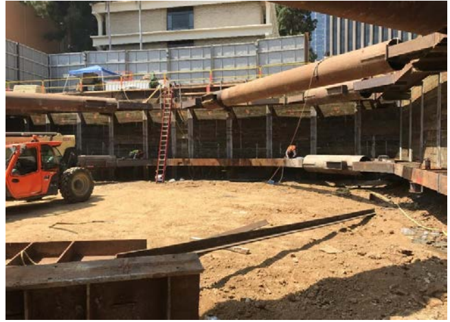
Tunnel Access Shaft Excavation in Century City
