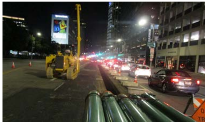
Southern California Gas Installation of Main Line A on Wilshire Blvd.
