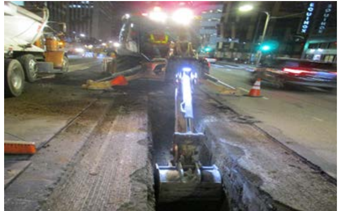
Southern California Gas Excavation and Potholing at Station 14+00
