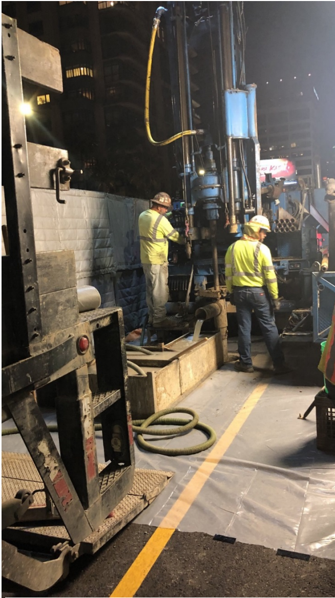
Geotechnical Boring for Cross Passage and Tunnel on Wilshire Blvd.
