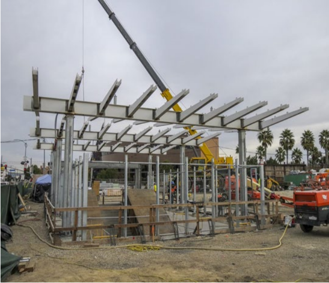
EXPO/CRENSHAW STATION – Canopy over main station entrance.
