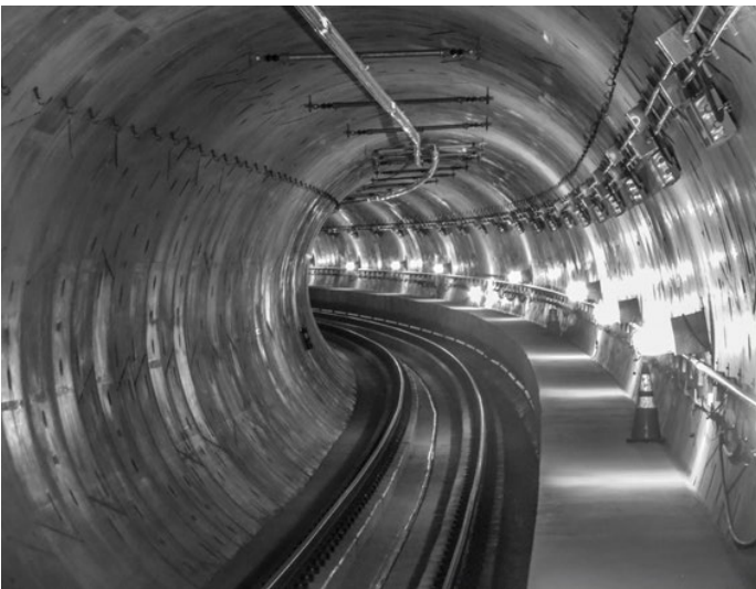
MARTIN LUTHER KING JR. STATION – Tunnel view leaving station.
