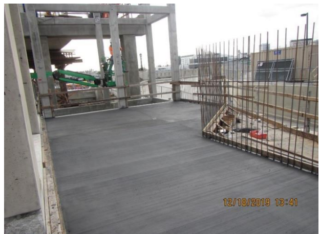
Elevator Platform, Poured
