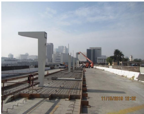
Bus Platform Canopy, Columns installation.
