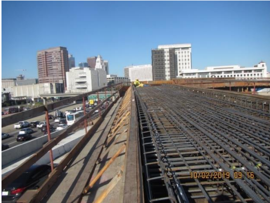
Pedestrian Bridge, Rebar/Electrical conduits
