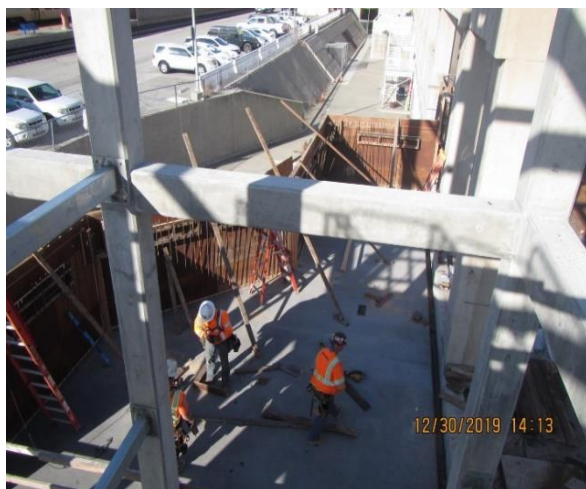
Elevator Platform, Forming the walls.
