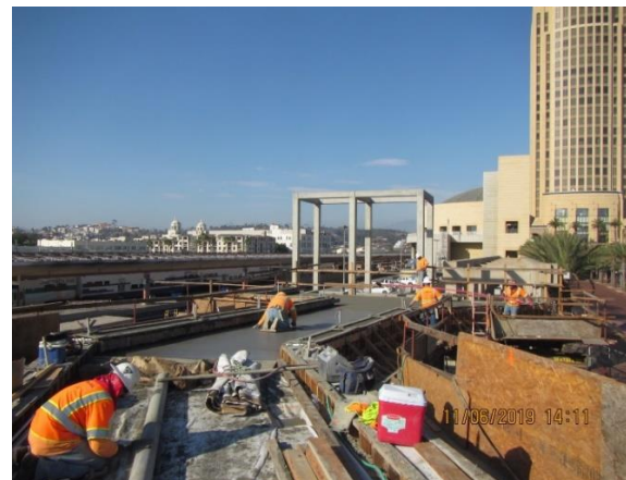
Pedestrian Walkway, poured
