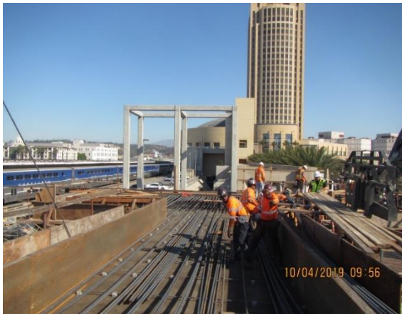
Pedestrian Walkway Rebar
