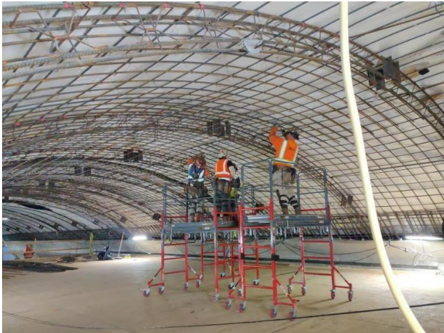
Rebar installation for crowns in SEM Cavern
