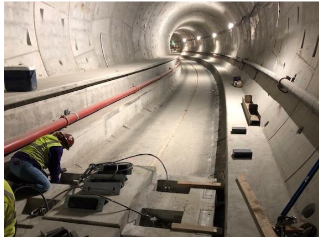
Floating slab installation in the left tunnel
