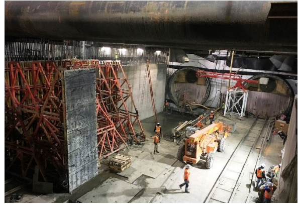
Wilshire/La Brea Station North Exterior Wall
