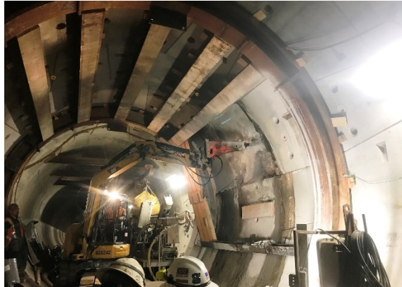
Cross Passage 10 Construction
