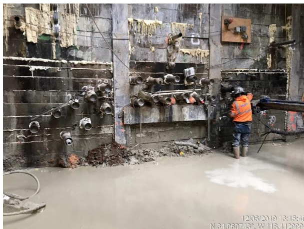
Canopy Pipe Drilling at the Tunnel Access Shaft in Century City
